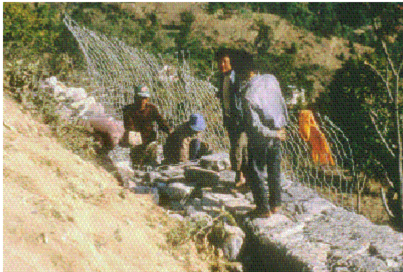
Check dam-Gabion
