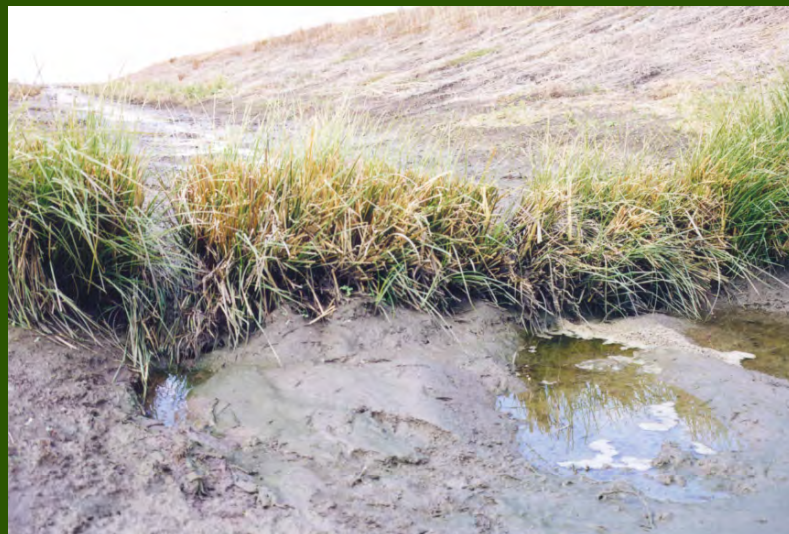
Vetiver strip trapped sediment
