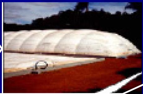
Pre-Project Activity Condition Anaerobic Digester with Co-gen Flare
