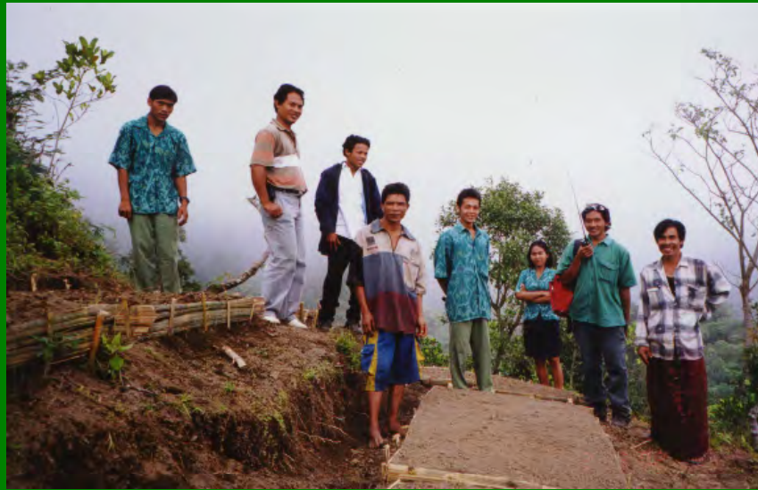
March 2002: terraces cuts in barren hills
