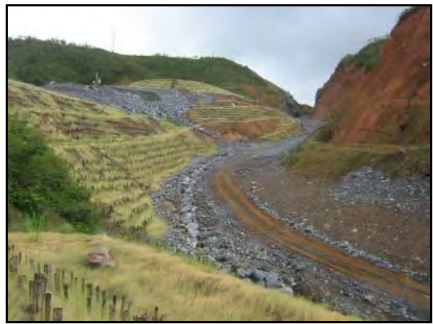
Ambatovy Pipeline project
