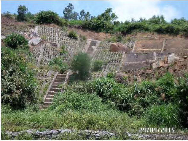
Collapsed section was repaired and planted with vetiver
