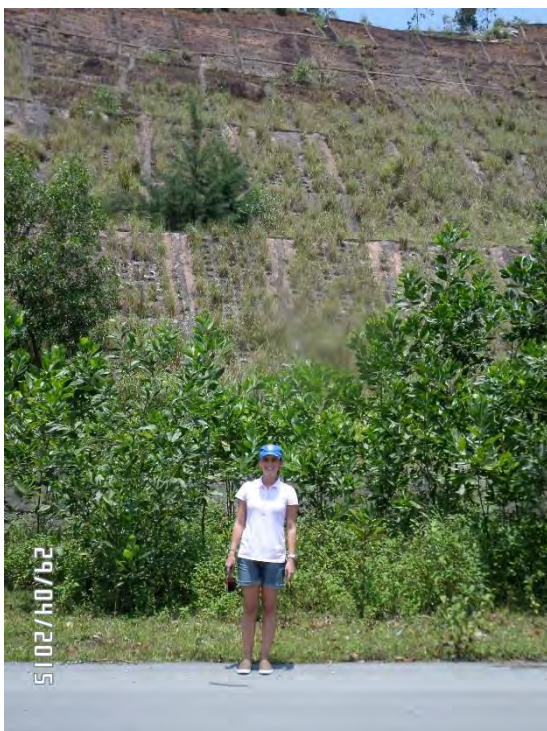
Vetiver planted in to the honey-comb concrete slabs to prevent them from slipping
