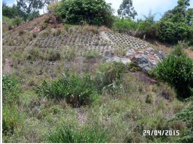
Collapsed section was repaired and planted with vetiver
