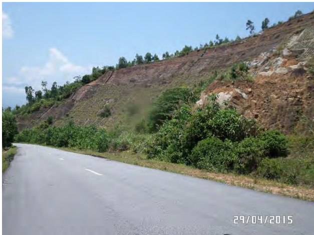
Honey-comb concrete slabs used to stabilise a very high and extremely erodible road batter.
