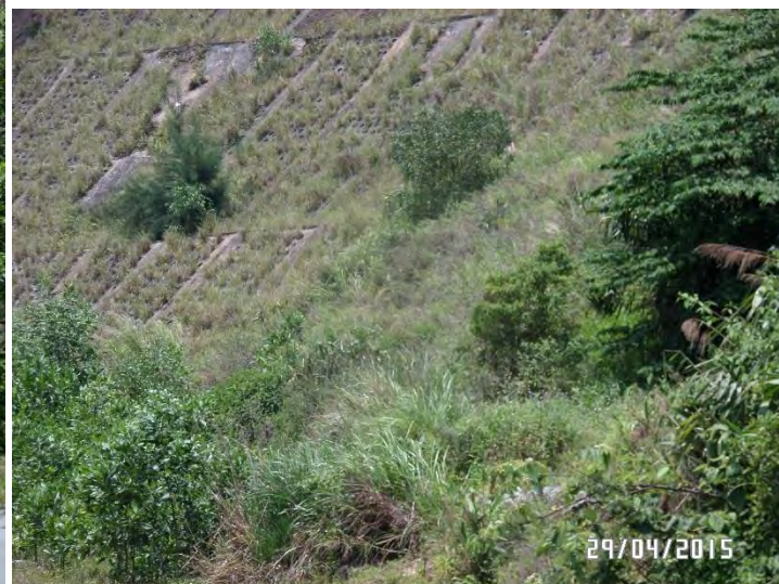
Vetiver planted in to the honey-comb concrete slabs to prevent them from slipping
