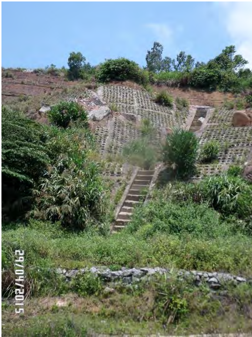
Collapsed section was repaired and planted with vetiver
