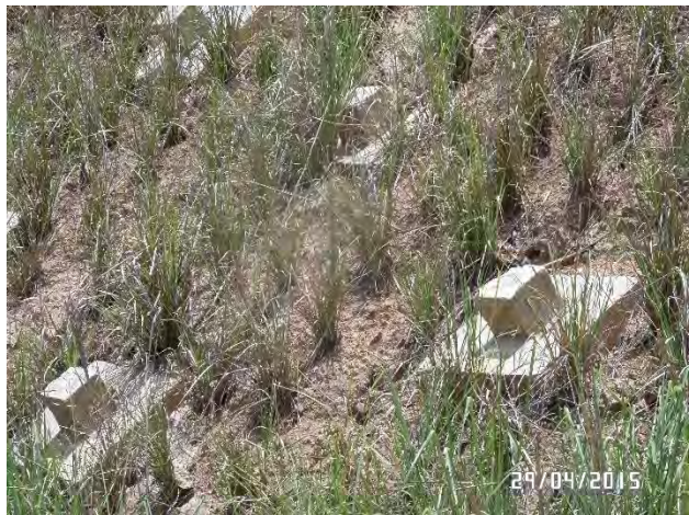
Planting on bare surface of soil nailed area to protect from surface erosion
