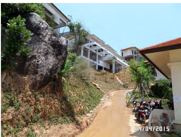
Planting on bare surface of soil nailed area to protect from surface erosion
