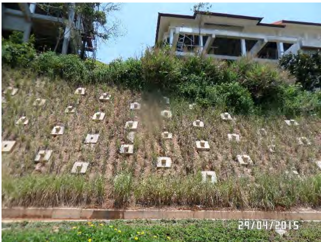
Planting on bare surface of soil nailed area to protect from surface erosion
