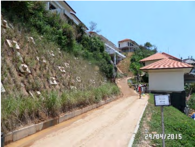
Planting on bare surface of soil nailed area to protect from surface erosion
