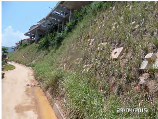
Planting on bare surface of soil nailed area to protect from surface erosion
