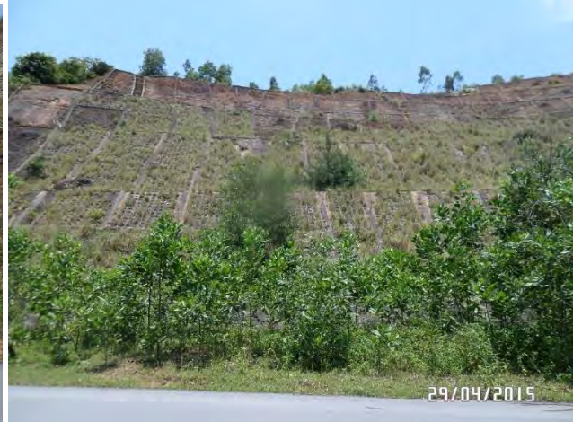
Honey-comb concrete slabs used to stabilise a very high and extremely erodible road batter.
