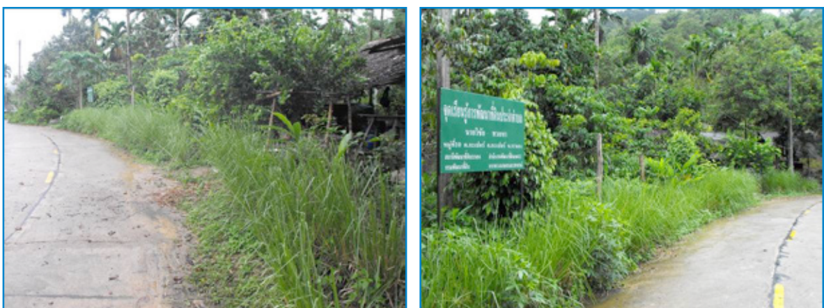
Figure 3 : Planting vetiver grass to protecting roadsides
