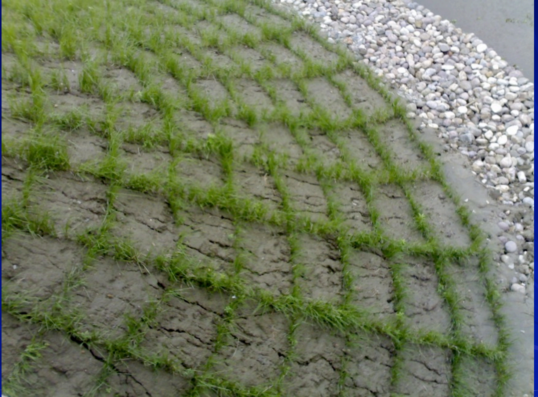
The forward slope with toe protection
