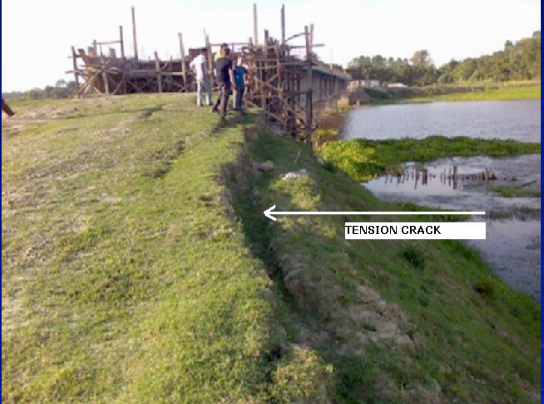
Doria bridge approach in Majuli; during construction
