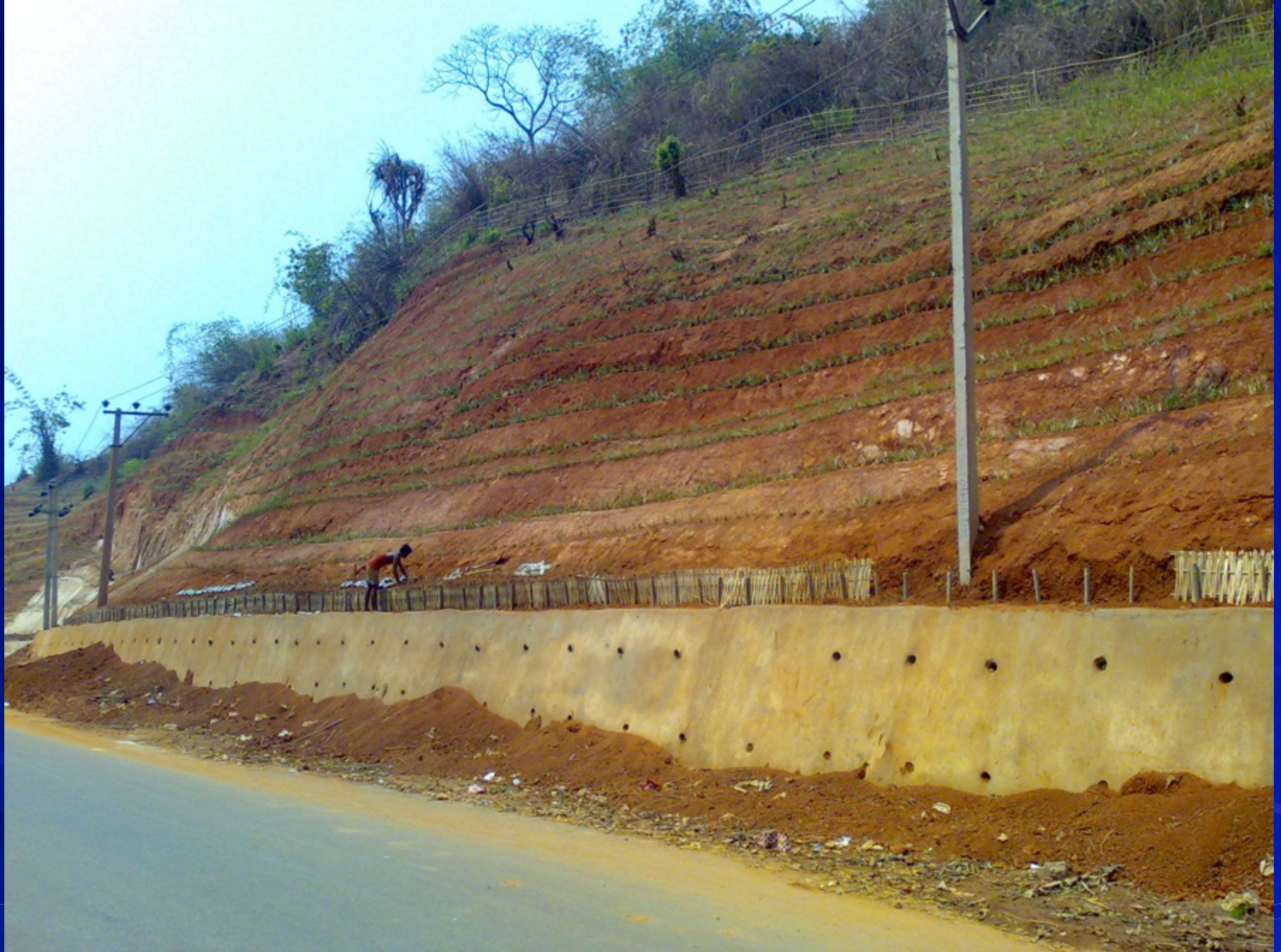
Plantation of Vetiver on the same slope
