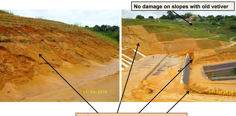
Several instances of damage on unprotected slopes and on slopes recently planted with vetiver
