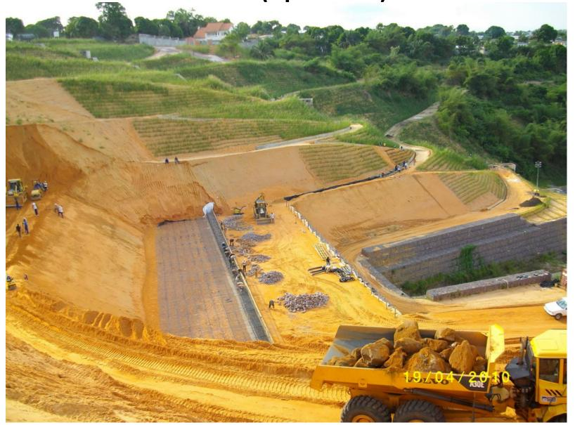
After rainfall events, the site has been damaged on several unprotected slopes and on slopes recently planted with vetiver, but no damage was seen on slopes protected with old vetiver.
