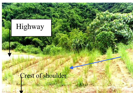
Figure 5 : Vetiver planting at steep gradient of highway shoulder to slow down runoff longitudinal.
