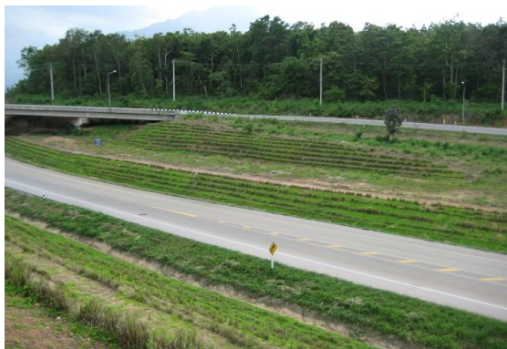
Figure 3 : Stabilization with vetiver along the stream bank.
