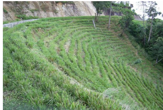
Figure 4: Vetiver planting at the side ditch lining.
