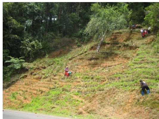
Figure 12 : Vetiver system was applied for stabilizing and stopping soil movement on highway slope ( Route No.1249 ).
