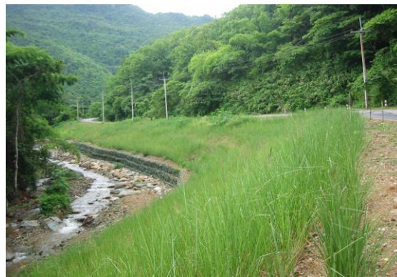
Figure 5 : Vetiver planting at steep gradient of highway shoulder to slow down runoff longitudinal.
