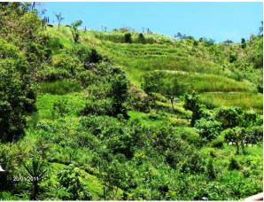
This effective slope stabilization and the mulch reduced sediment runoff provides a real life testimony for Vetiver which thus far remains in great condition. The ultimate test on January 11 and 12, 2011, when after an initial 18 mm it rained 95 mm
