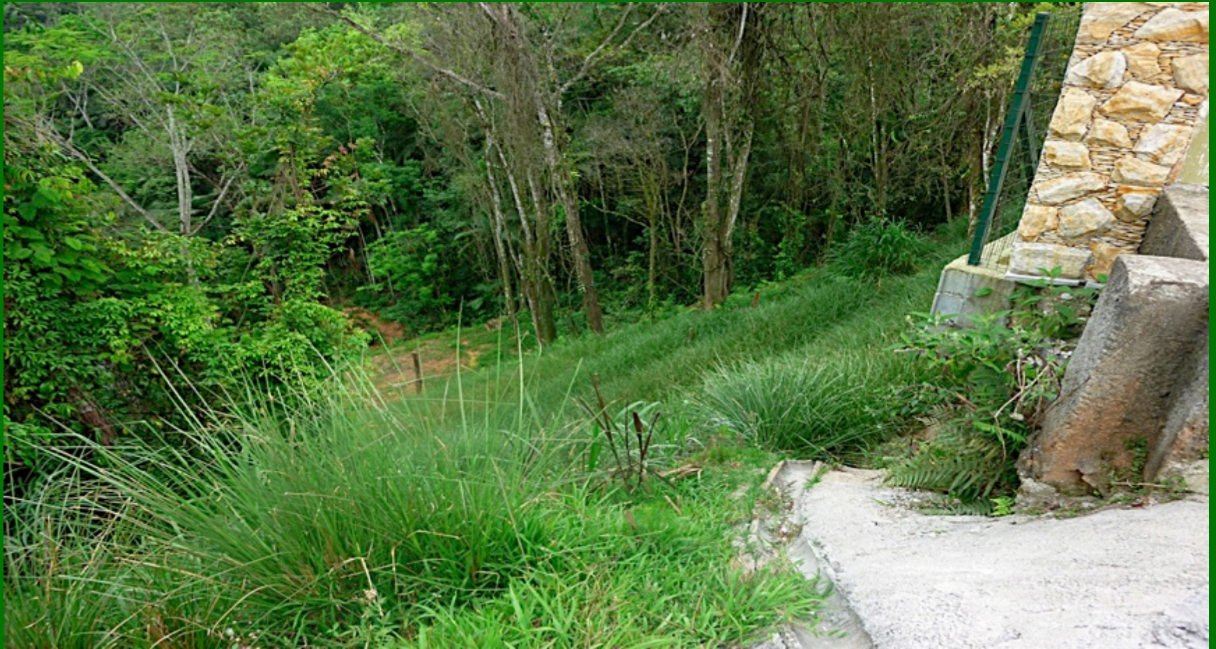
Brazil – Residential Slope Stabilization
