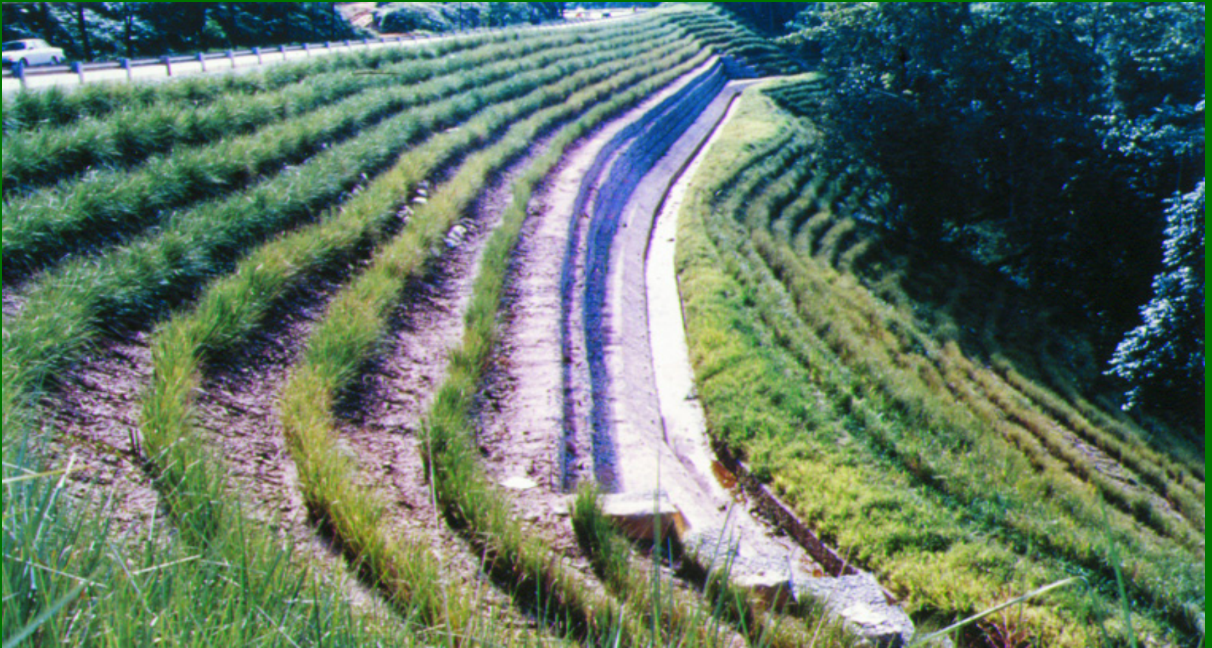
Malaysia – Highway Stabilization
