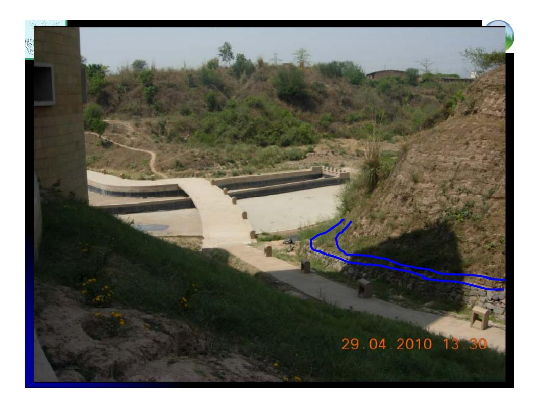
Rows of vetiver @ 7plants/m, rows at 1m spacing quantity as per measurement at site
