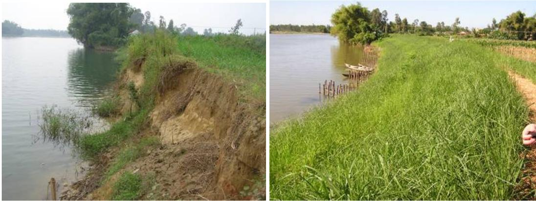
**Photo 6:** Stabilisation of a large river bank against flash flood erosion
