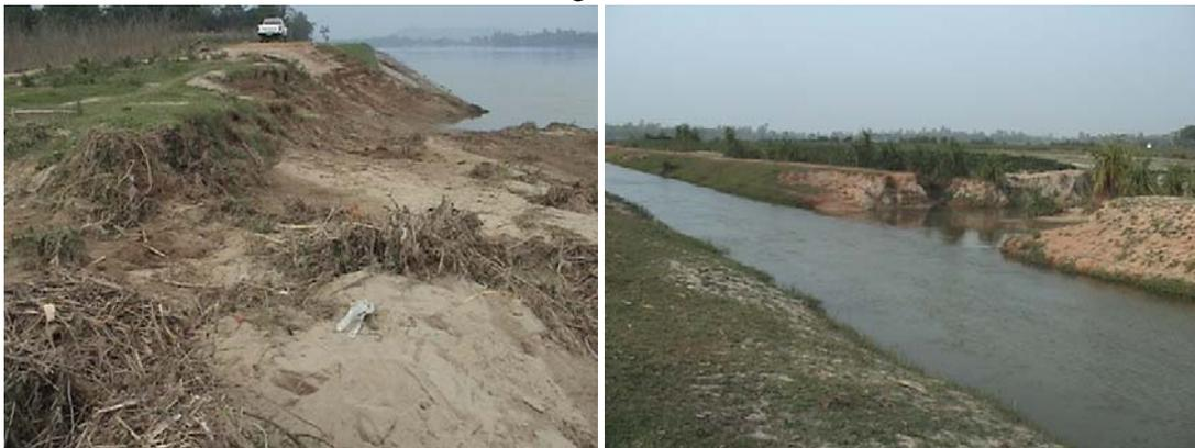
**Photos 2:** Flood damages to irrigation channel and farm dike
