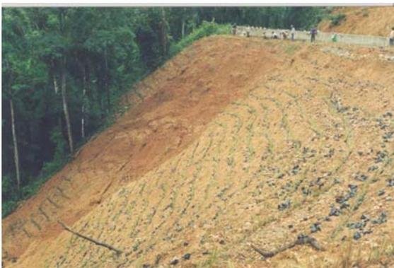
Fig.16 Shallow seated failure of embankment slope at STA.15+325-STA.15+510L before stabilized by vetiver.
