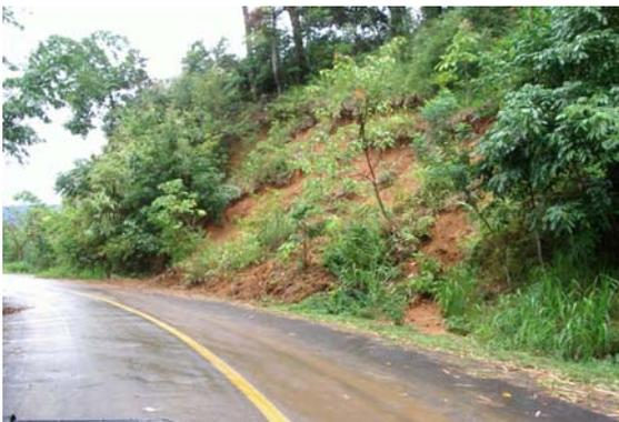
Fig.4 Erosion and shallow seated failure on highway cut slope
