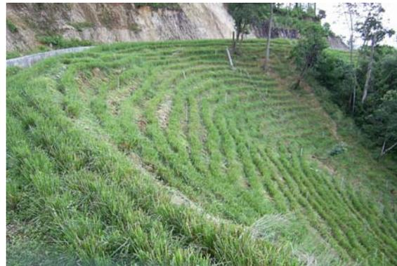
Fig.17 Repair of the collapse embankment slope in Fig.16 and stabilized with vetiver.
