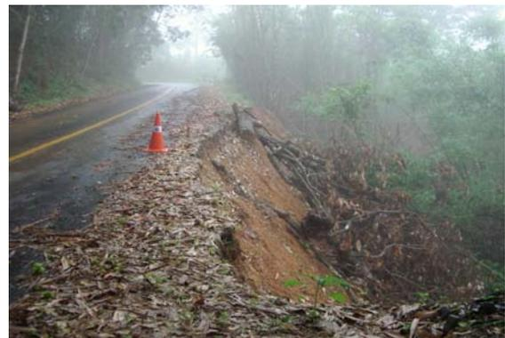
Fig.5 Shallow seated failure on highway embankment slope
