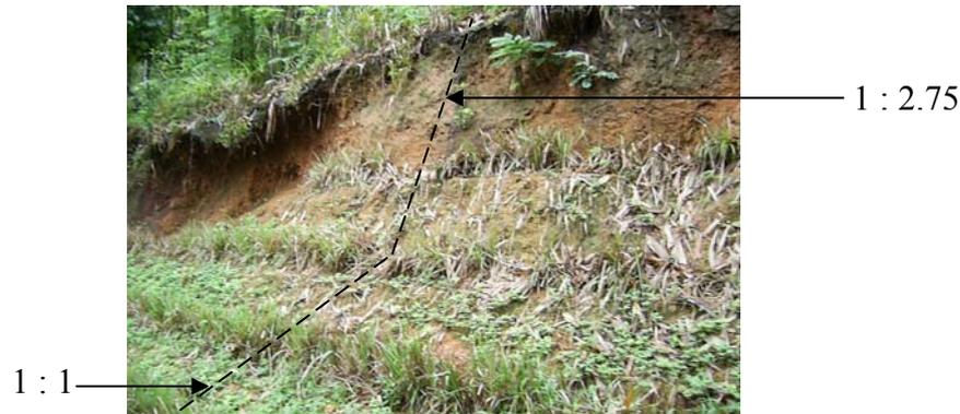
Fig.15 Difference growth situation of the vetiver planted in steeply ( $>70^{\circ}$ , 1:2.75) and gently ( $<45^{\circ}$ , 1:1) inclined slope portions.
