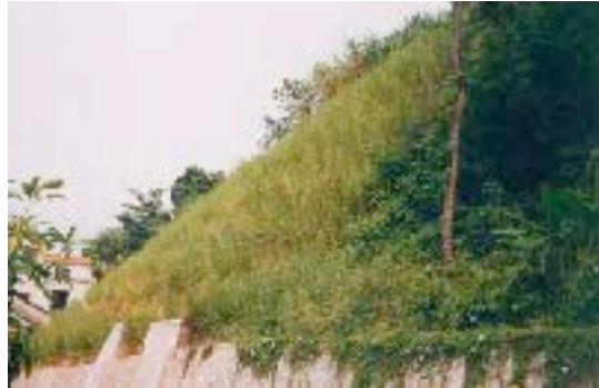
Photo 4 After the Eco-engineer of Vetiver in Nanyangxiang Slope, Zhongshan
