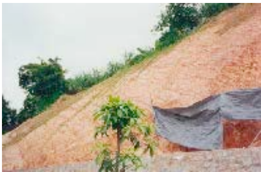
Photo 3 Before the Engineering of Nanyangxiang Slope, Zhongshan
