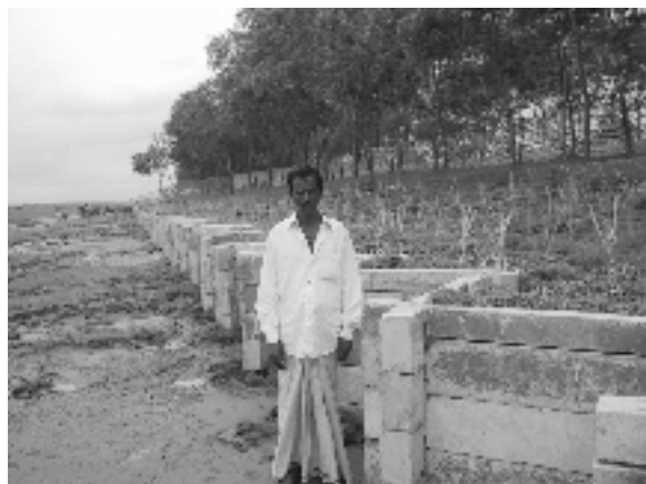
Fig. 7 Toe protection trial by zigzag RCC beams (June 02)
