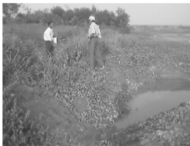
Fig. 3 Vetiver planted at the seaside toe line
