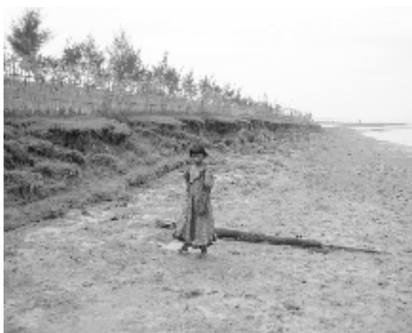
Fig. 2 Creeping toe erosion
