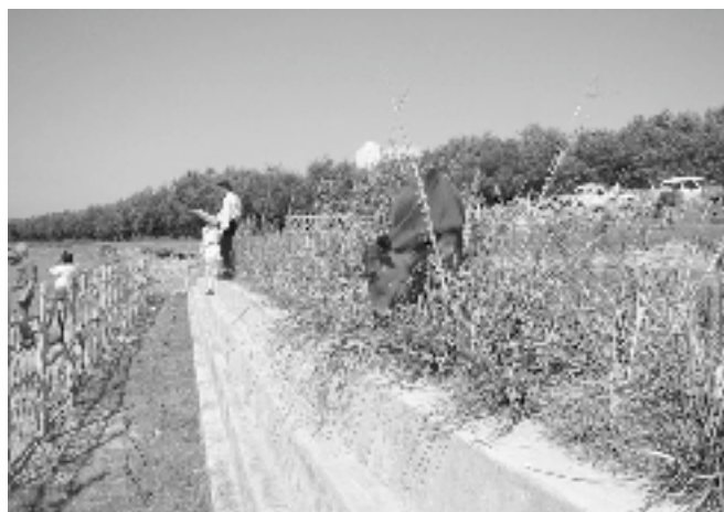
Fig. 6 Vetiver grass on Concrete Frame- toe protection wall
