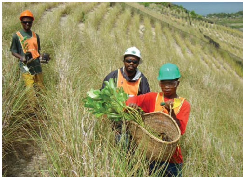
BELOW RIGHT: Good cover has been achieved with the hydroseeded grasses, after the initial stabilisation with Vetiver.
