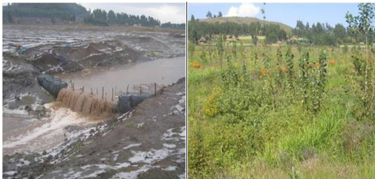
Plate 7. A gabion check-dam filled with soil (top and bottom plates) and its effect after one year
