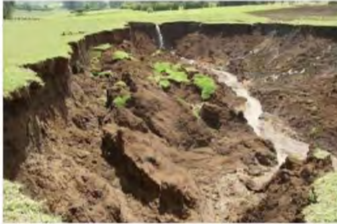
Figure 6. Effects of soil erosion in the study area
