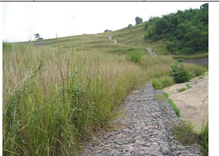
2. Same site one year later totally recovered and stabilized with vetiver grass
