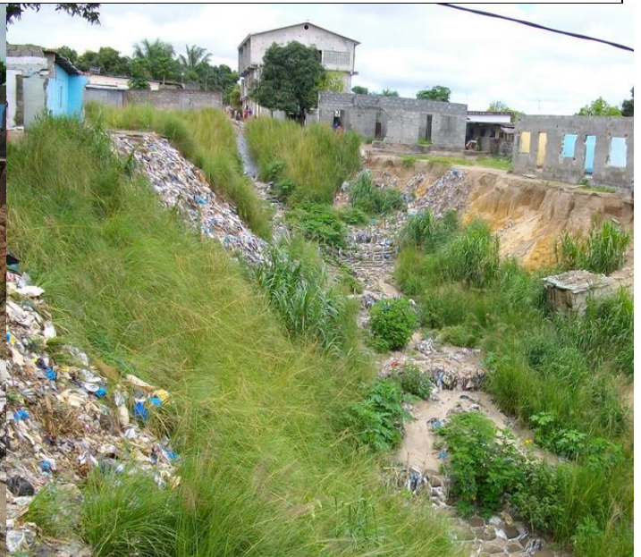
4. Same gully totally stabilized and stopped after planting vetiver , november 2009
