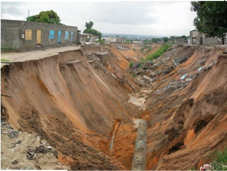
1. Initial state of Boukeni gully , february 2009
