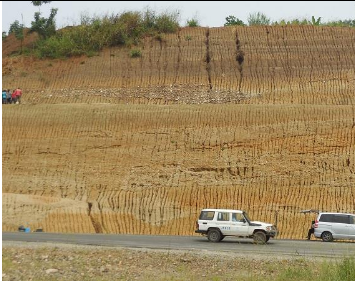
Initial status : Some erosion occurs on unprotected slop, august 2013
