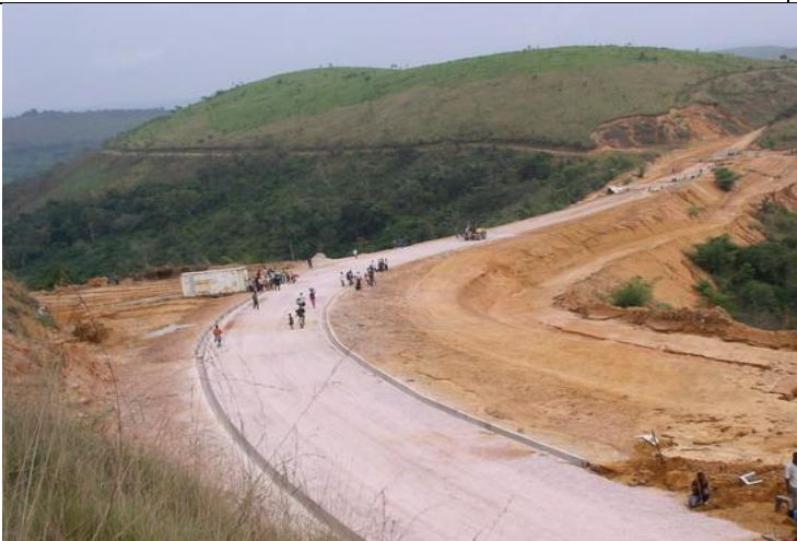
1. Fill embankment before vetiver planting, september 2007
