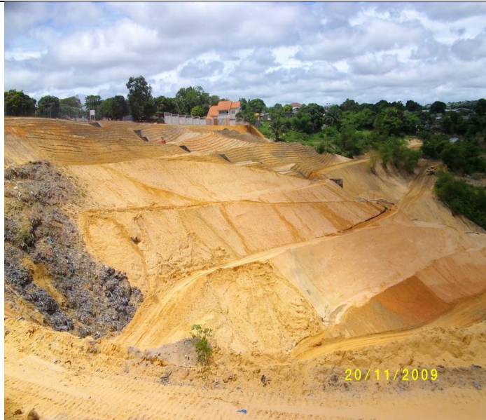
1. Casis erosion control project at Congo Brazzaville, november 2009
