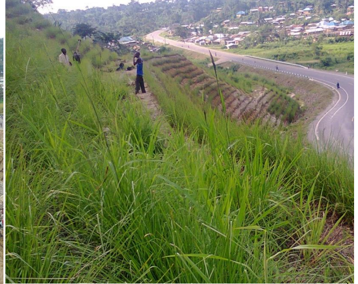
Ten months later, steep slope totally recovered and stabilized by vetiver grass, may 2014
