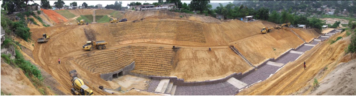
1. Hard structure work and planting vetiver in progress at Boukeni 2nd project, november 2012
