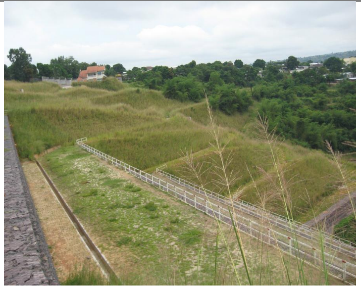
2. Same site completely stabilized, some months after planting vetiver
