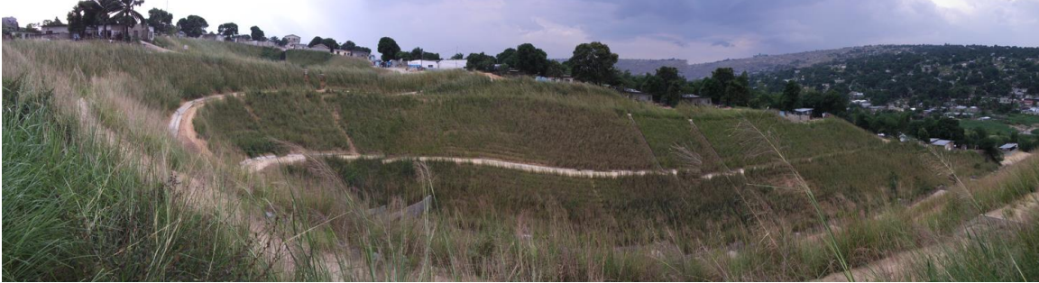
2. Same site totally stabilized, may 2014
