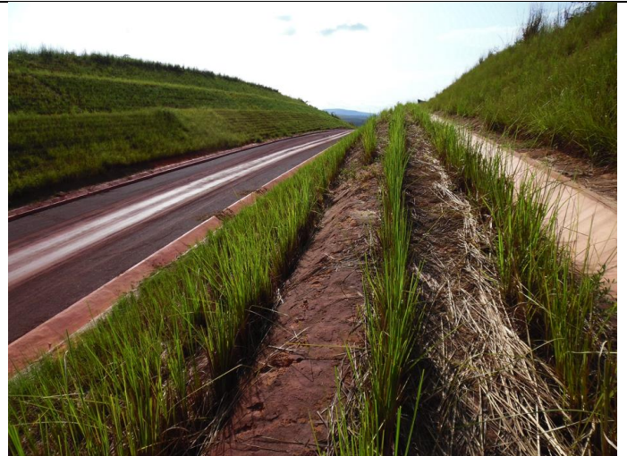
Road slope totally protected by vetiver grass, some months later
