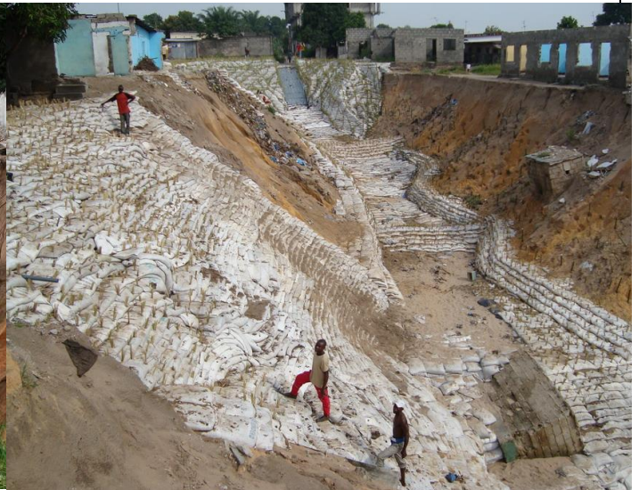
2. Placing sand bags and planting vetiver
