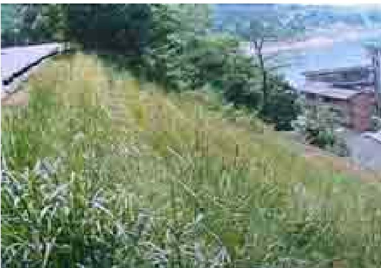
Collapsed highway stabilized with vetiver
