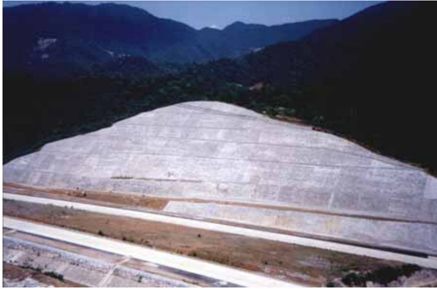
Fig. 11 A section of highway being constructed in northern hilly region of Guangdong. The huge up-slope is covered by cement wall that is very expensive and short of ecologic benefit.
