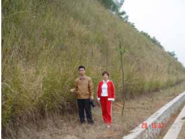
Fig. 19 The appearance of the section of up-slope of the Highway a year and a half after planting vetiver
