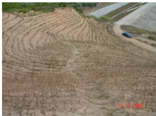
Fig. 25 Due to abnormal heat and subsequent long drought, vetiver grew very poor in winter, and other species all dies out in spite of the fact all plants were prepared with polybags and watered 1~2 times per day
