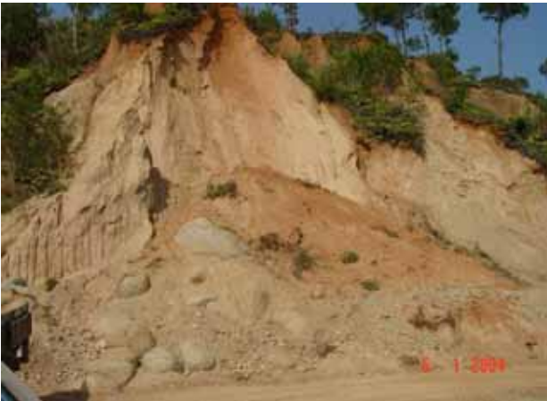
Fig. 23 Another slope of the reservoir assuming severe landslide, which would also be reined with the vetiver eco-engineering
