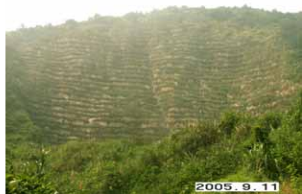
Fig. 33 Another completely different landscape exhibited in front of us after the complex vetiver eco-engineering was finished for 4 months
