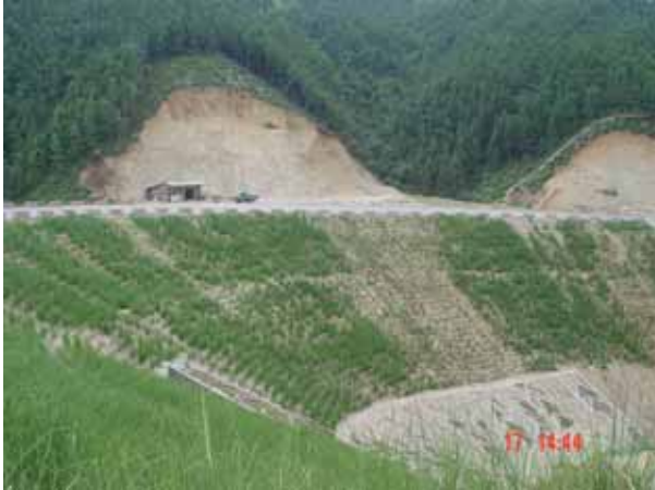
Fig. 18 The appearance of the section of down-slope of the highway two months after planting vetiver
