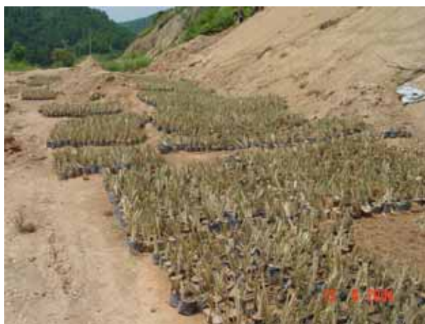
Fig. 24 Parts of vetiver seedlings, prepared in polybags on the spot, ready for the project of Wusijiang Reservoir slope stabilization
