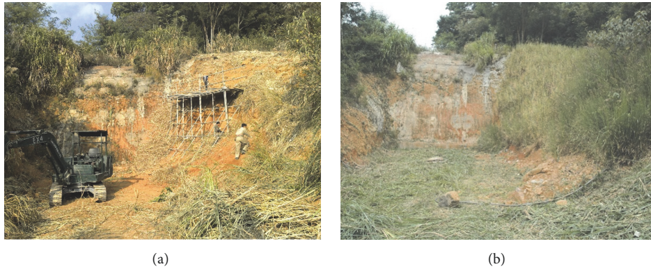
FIGURE 3: Panorama of research site (a) before grass planting and (b) during field testing.
