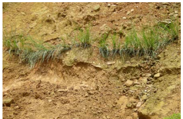
Vetiver stopped slope slide.
