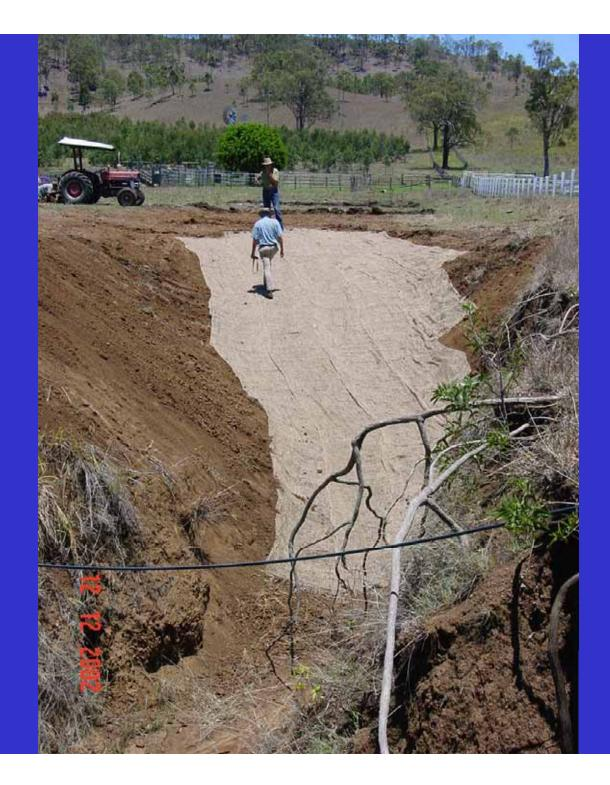
Cover with open jute mesh geofabrics
