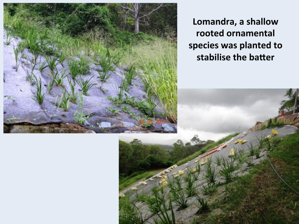
Despite this costly measure the batter collapsed during an average summer rainfall and it was rebuilt with imported fill materials
