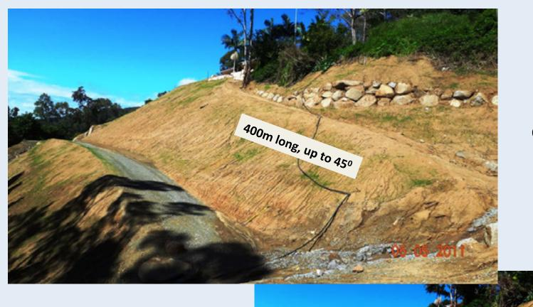
Original batter from material excavated and pushed down slope
