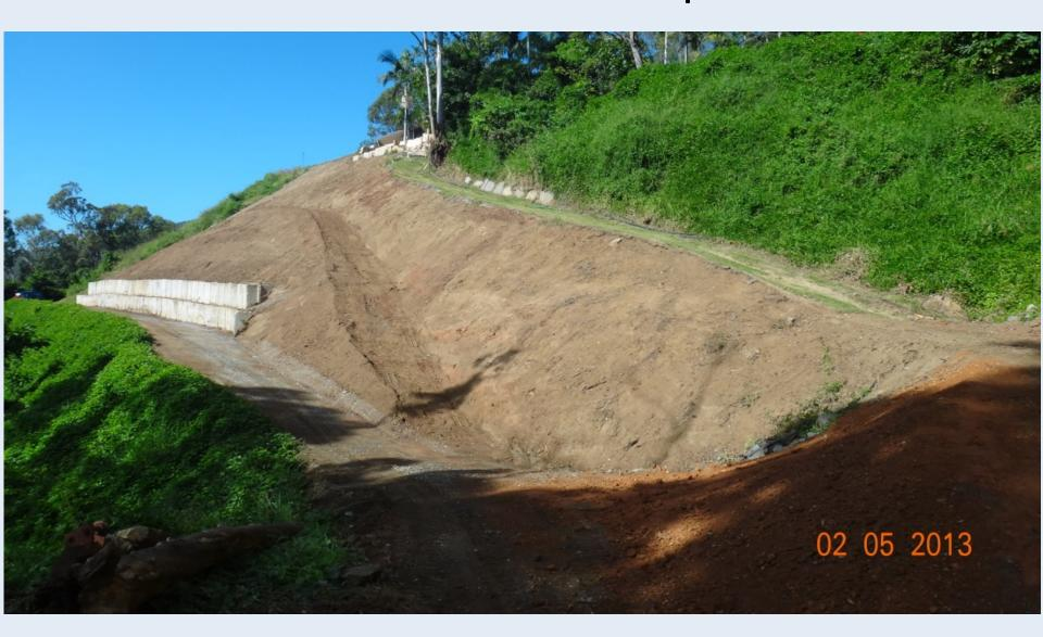
The batter was rebuilt with imported fill
