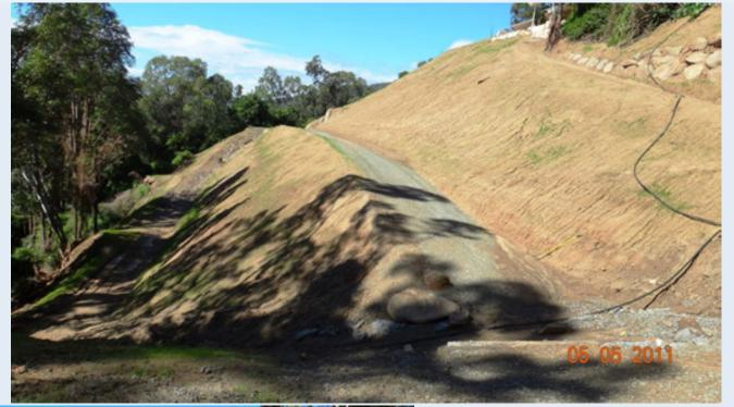
Highly erodible sandy soil with gradient up to 500 at some sections
