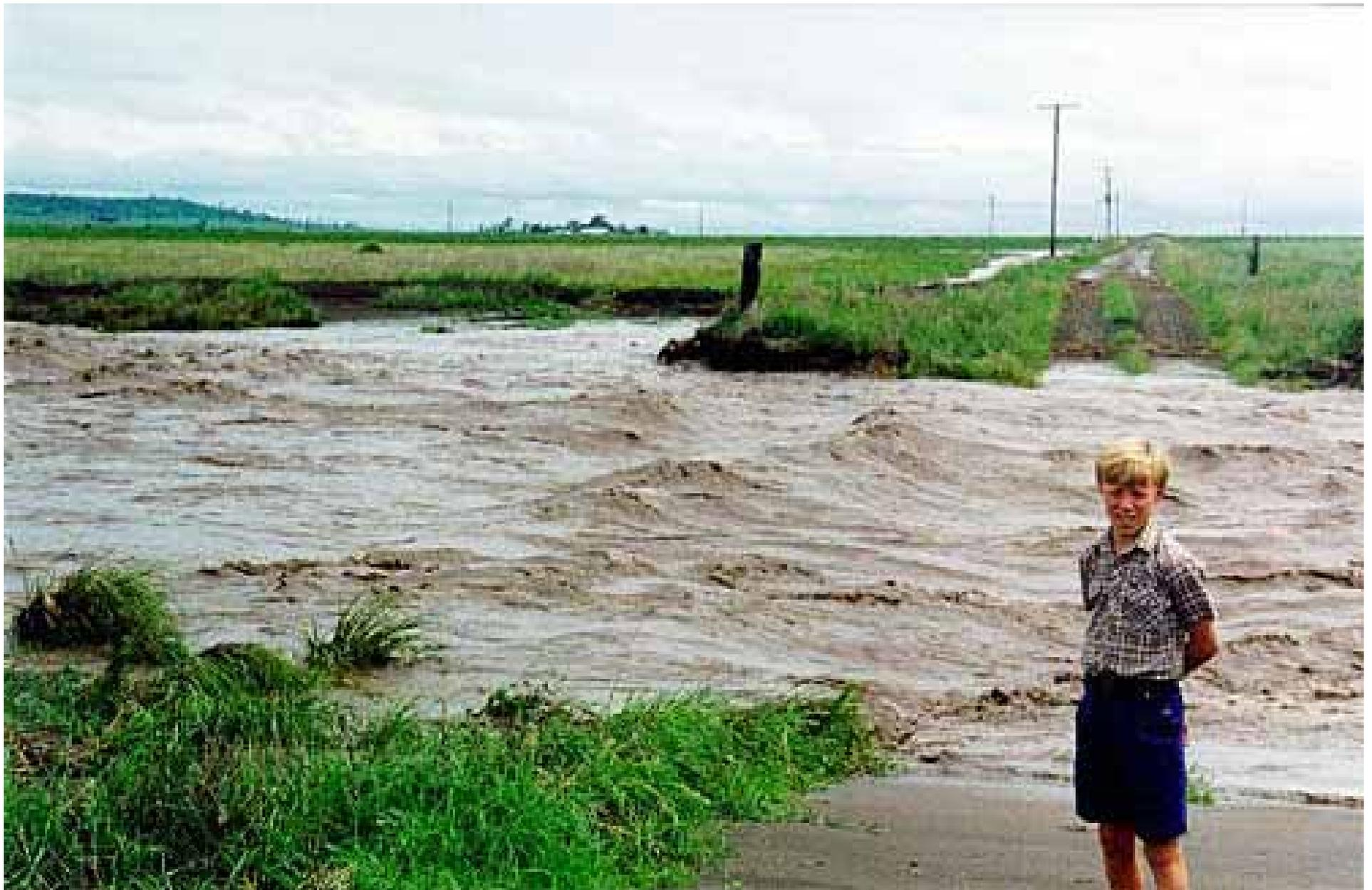
Although badly battered, the vetiver hedges held firm during the flood, preventing the undermining of the concrete causeway
