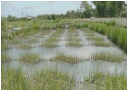
Wastewater effluent polishing (China)
