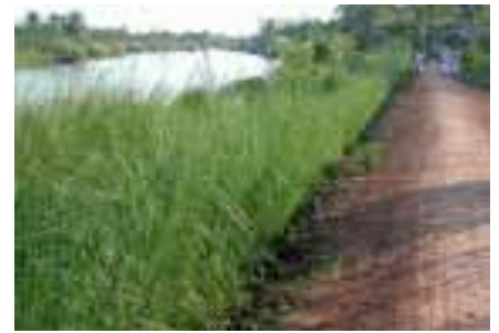
Canal bank protection (Viet Nam)
