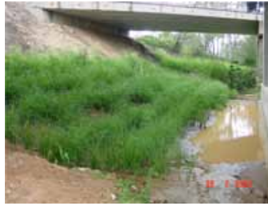
Bridge protected by vetiver hedges
