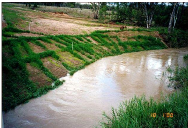
Figure 13. Vetiver planted on this streambank in Australia helps to stabilize it.
