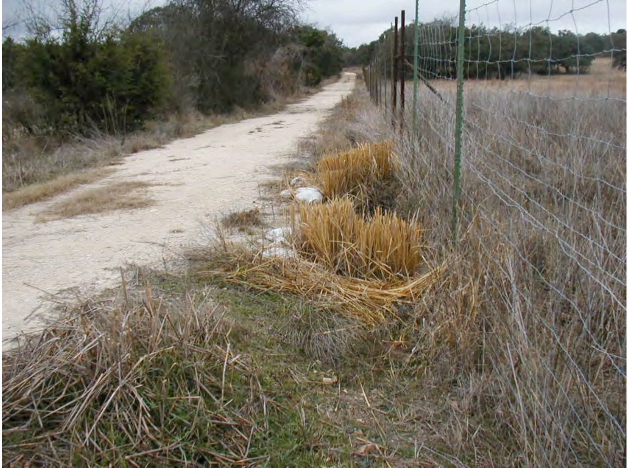
Photo 4. Vetiver planted to protect soil : concrete interface of culvert and to take velocity out of runoff in the road drains.
