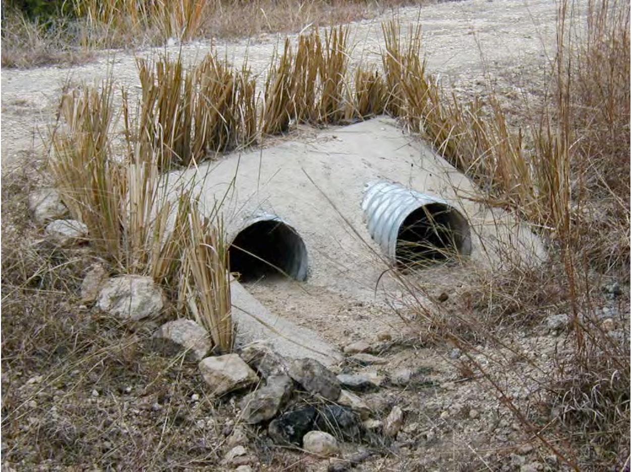
Photo 7. Another culvert that we have protected with vetiver.
