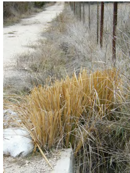
Photo 4. Vetiver planted to protect soil : concrete interface of culvert and to take velocity out of runoff in the road drains.
