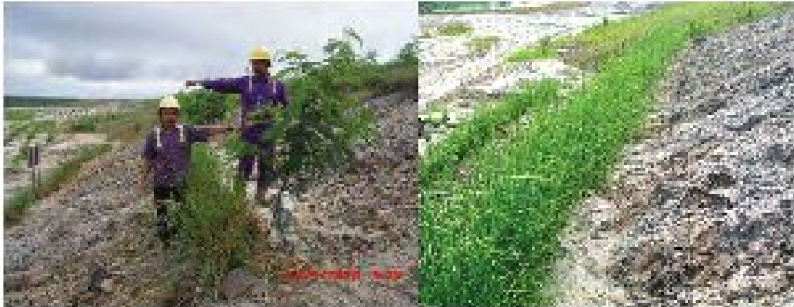
Figure 58. Sediments trapped by Vervet after only 4 months after planting. Source: www.ecoliva.org
