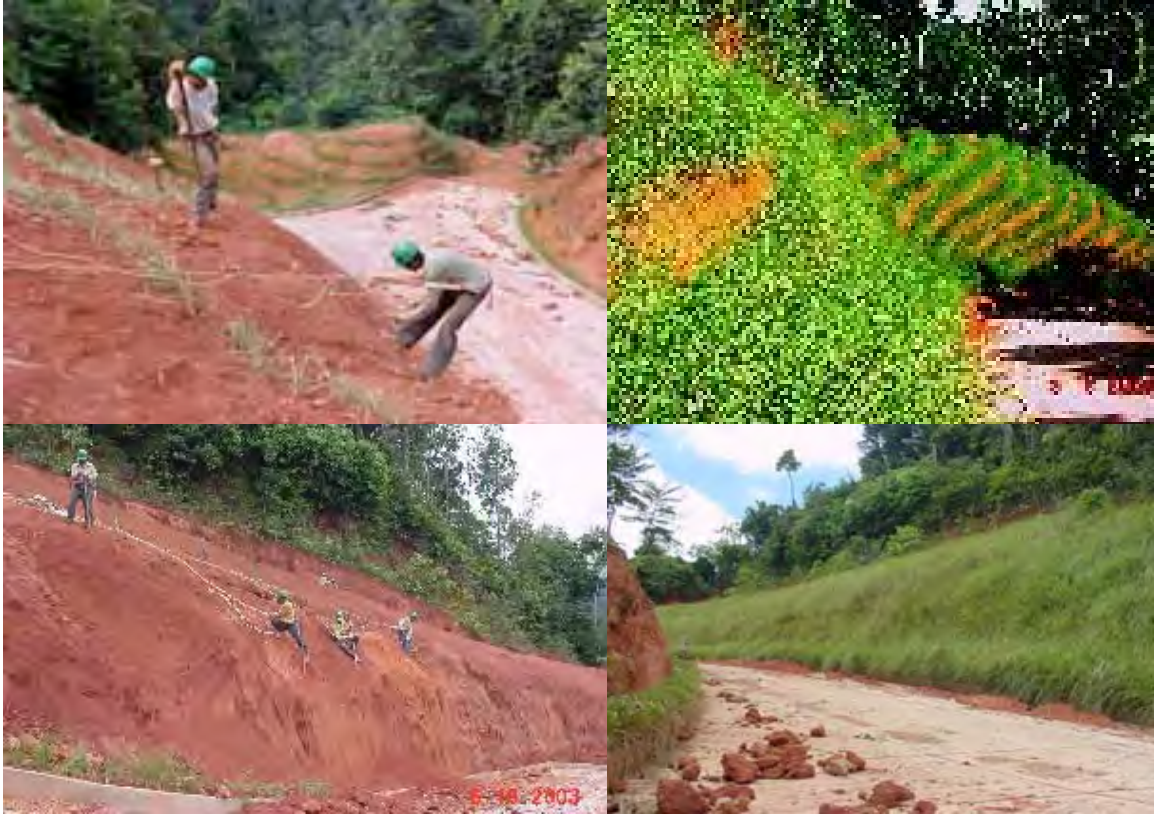
Figure 63. Various slopes (left) stabilized by Vetiver (right). Source: Luque et al., 2006.
