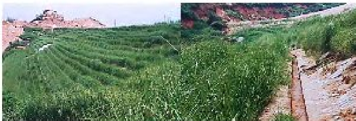
Figure 41. Vetiver planting on the slope of this old landfill mound in Guangzhou (left). leechate seepage was completely stopped one year after planting (right).
