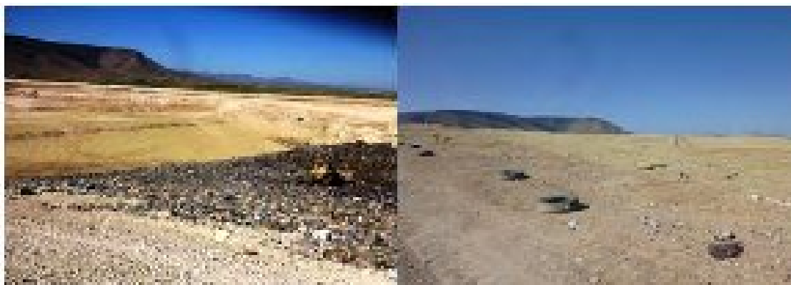
Figure 37. Fresh industrial and domestic wastes being compacted (left) and site ready for Vetiver planting (Etienne Richards, pers.com.).
