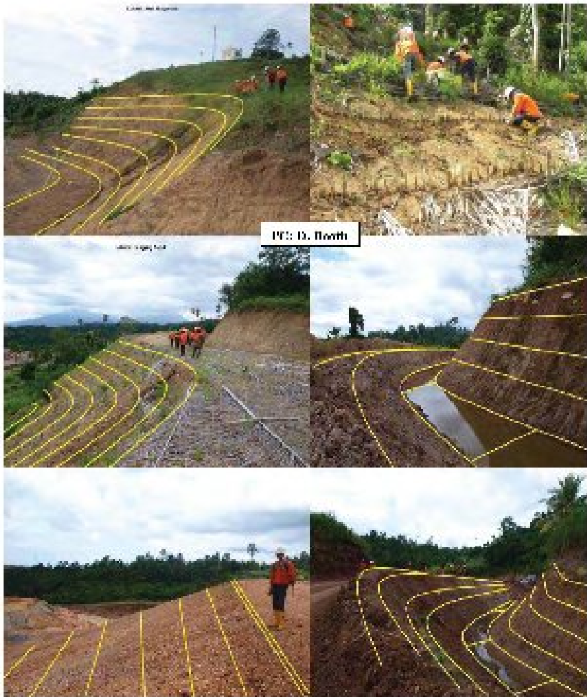
Figure 48. Design and application of vetiver grass technology throughout extensive infrastructure and drainage. Source: www.vetiver.org
