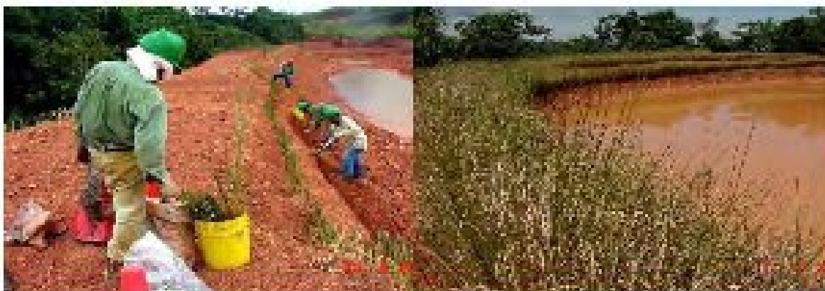
Figure 65. Vervet planted for reinforcement of lagoon dikes (left) and 14 months after planting (right). Source: Lague et al., 2006.
