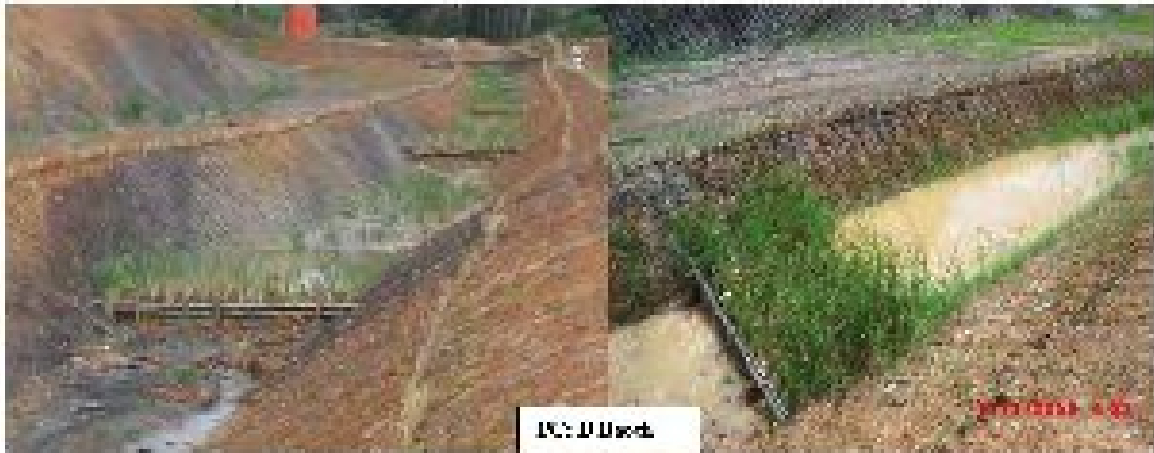
Figure 59. Vervet planted for channel bank stabilization (along the channel) and sediment traps (across the channel). Source: www.ecoliva.org
