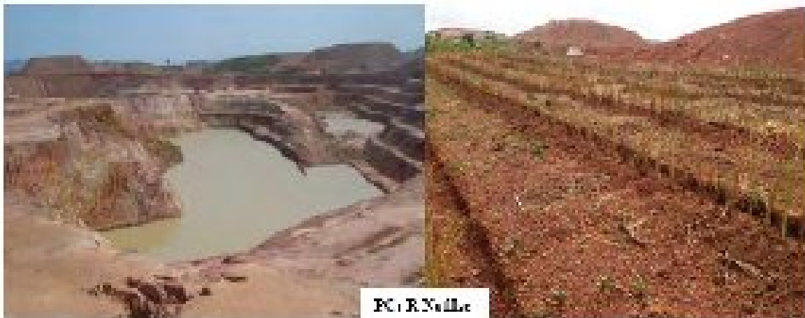
Figure 51. Vetiver application at Anglo American gold mine in Guinea, West Africa. Source: Nollke, 2013.
