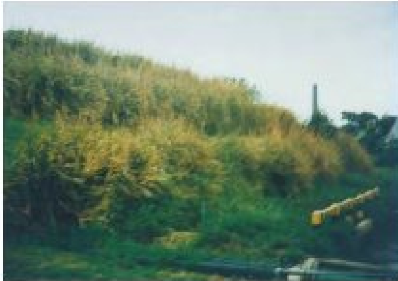
Figure 50. The same gold mine tailings dam after three years of Vetiver cultivation (Tony Tatum pers.com.).
