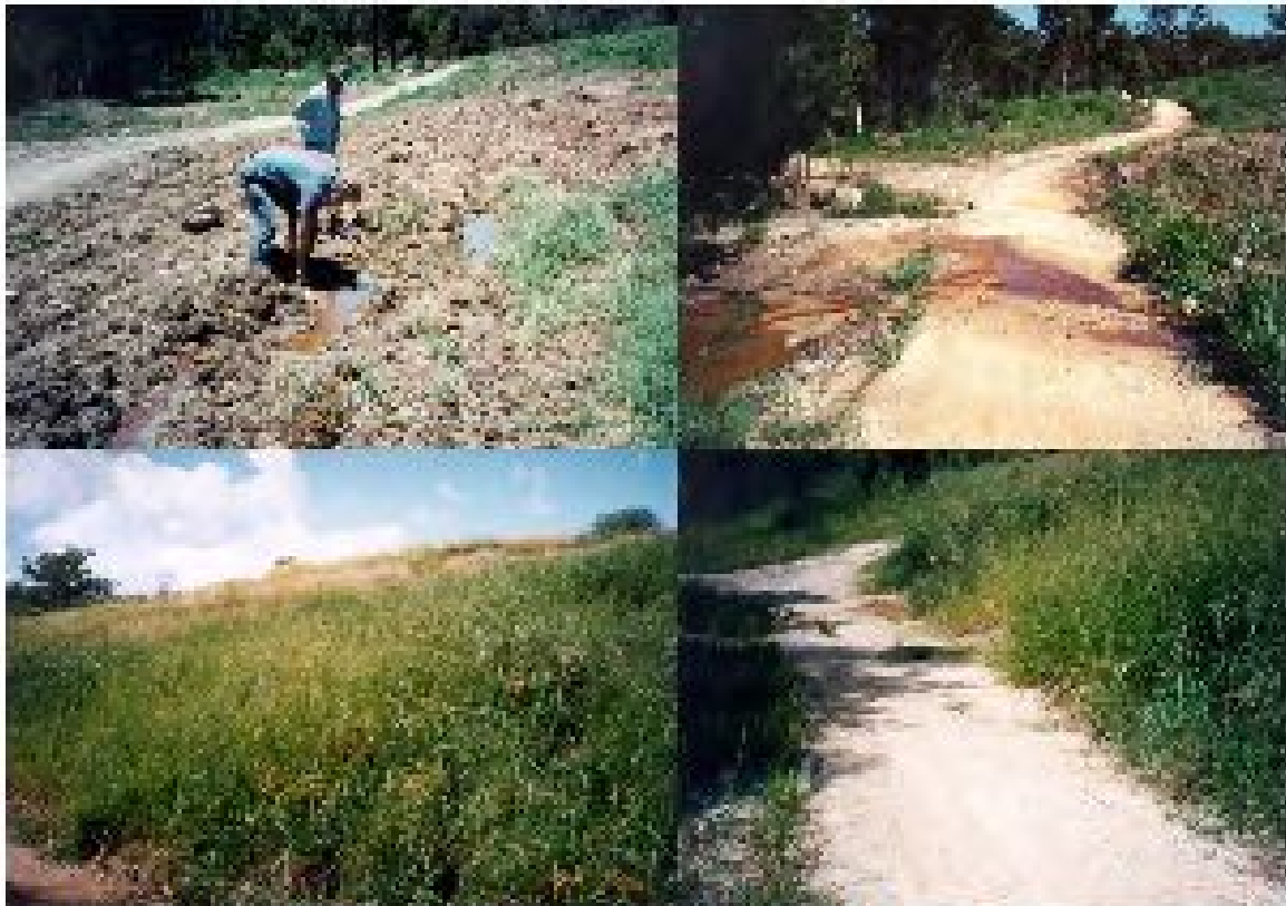
Figure 40. Leachate after rain on the side slope of the old landfill mound (top), within a year Veriver completely stopped the leachate seepage (bottom)
