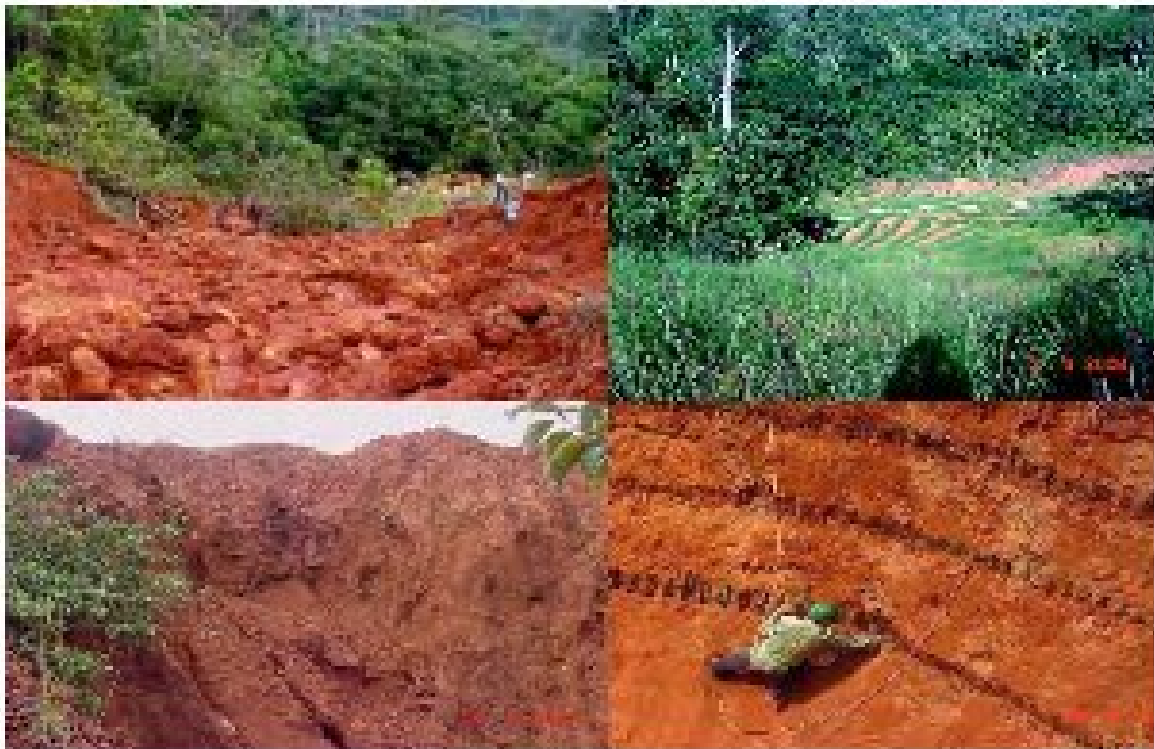
Figure 64. Gullies (left) stabilized by Vervet grass (right). Source: Lague et al., 2006.
