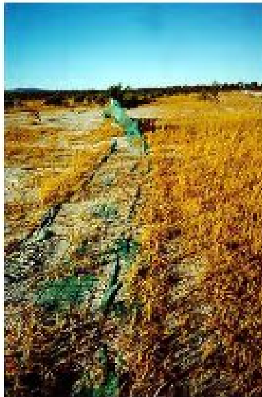
Figure 45. Despite its very solid construction, these rigid and expensive fences are also vulnerable to high wind velocity
