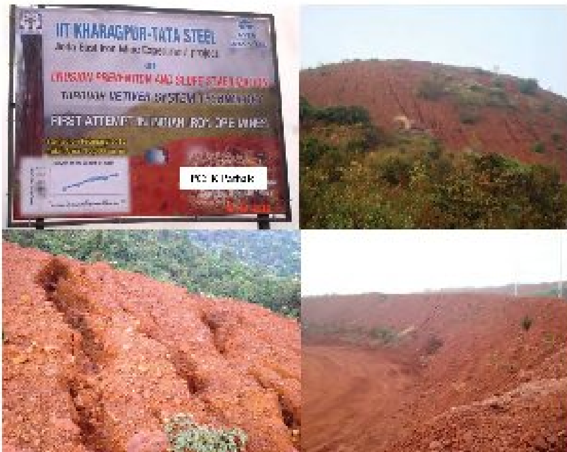
Figure 26. The old waste dump is highly erodible and steep (top and bottom left), and re-shaped to 40 (bottom right).
