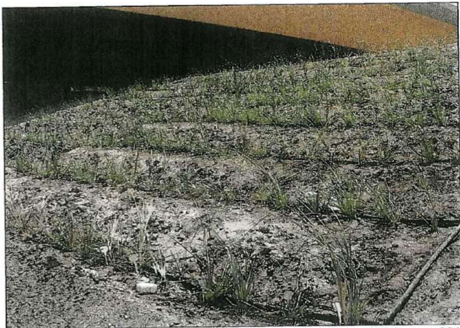
Plate 4. Overview of the roadway embankment site at Surra (15 August 2011).
