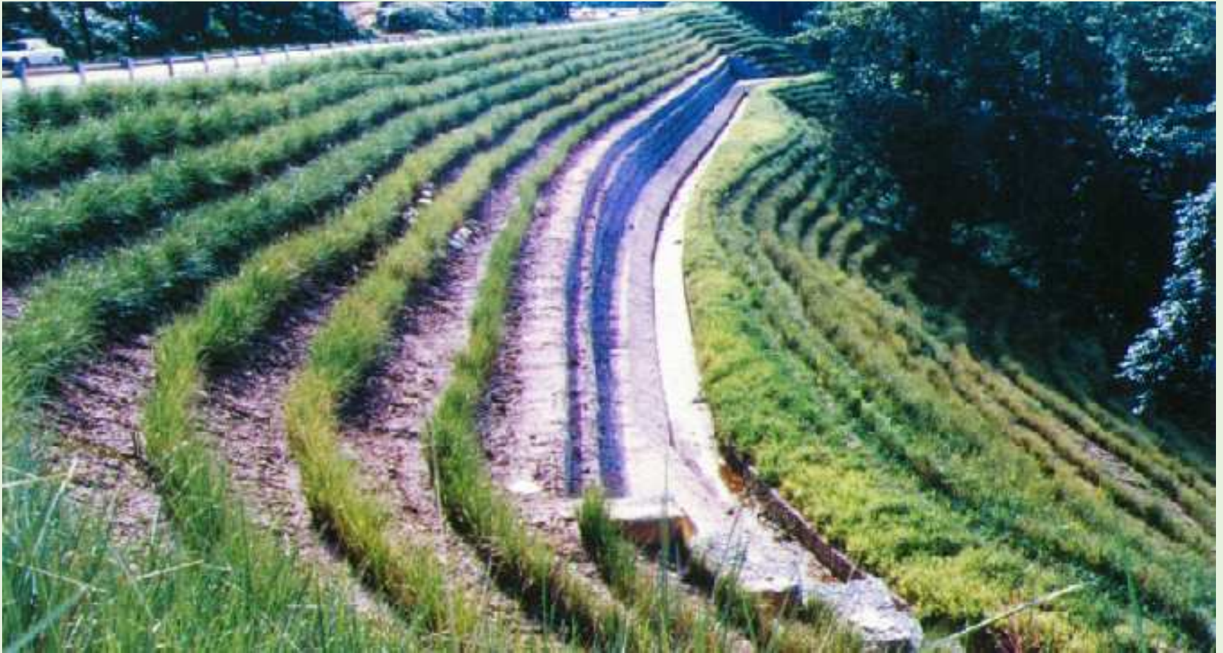
Malaysia – Highway Stabilization
