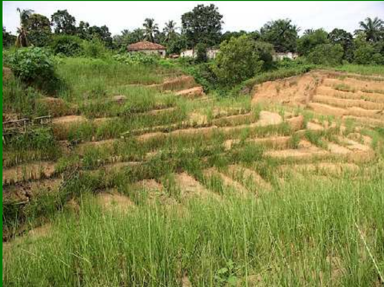
Gully stabilization in the Congo (DRC)
