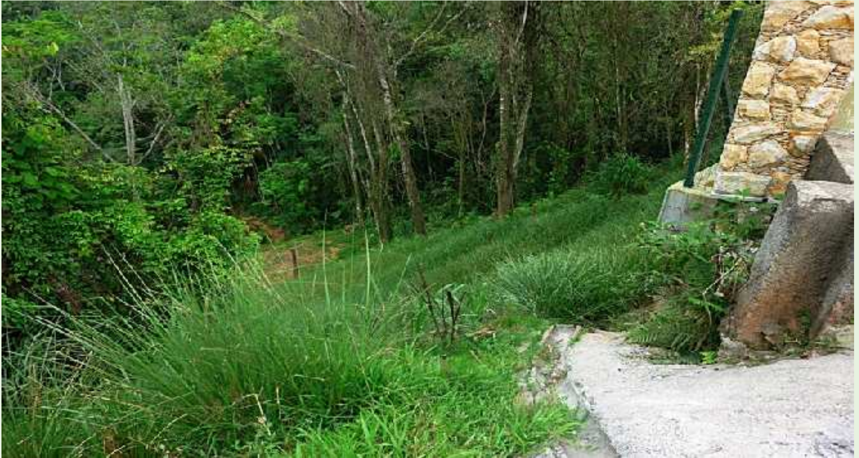
Brazil – Residential Slope Stabilization
