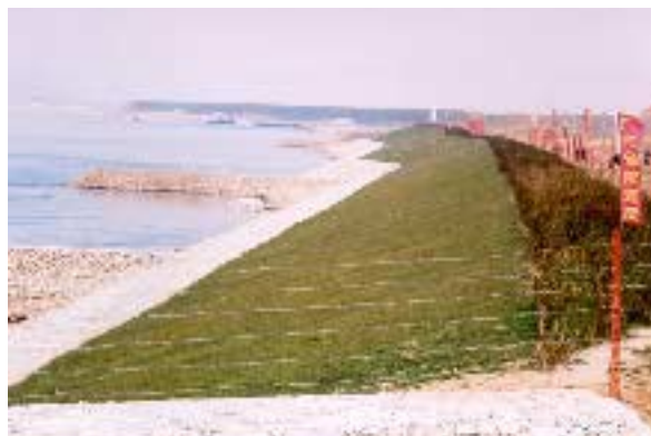
Stabilisation of the Pearl River bank at San Shui
