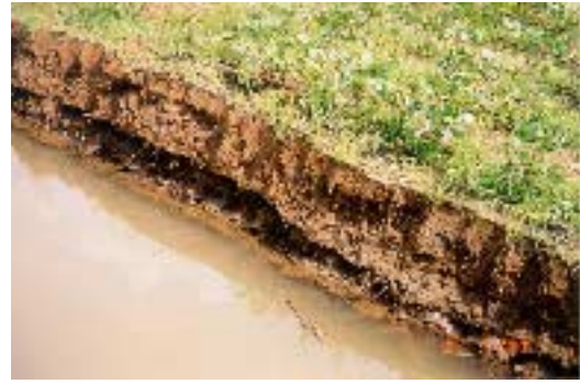
Erosion on the bank of the Mekong
