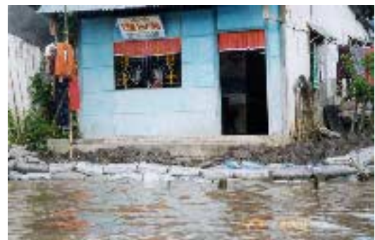
Erosion on the bank of a tributary
