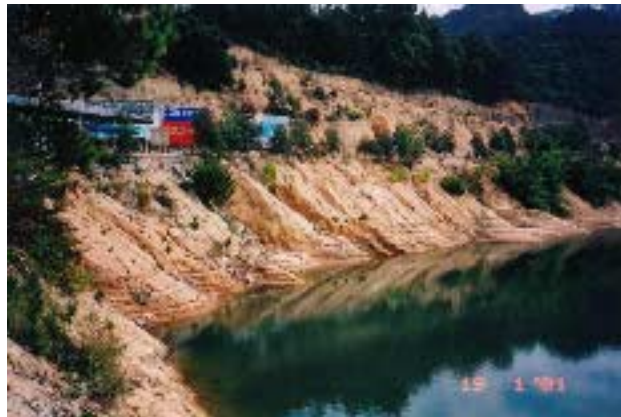
Badly eroded shoreline of the Evergreen Lake in Heyuan
