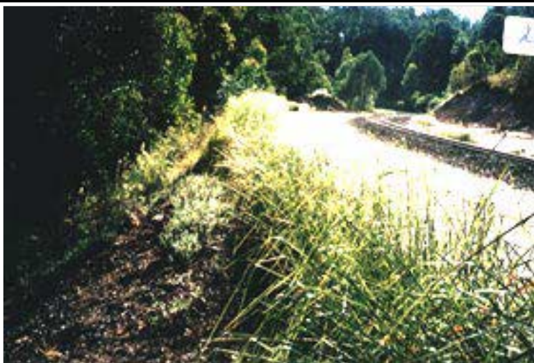
Australia: Railroad embankment stabilized with vetiver grass hedgerows. Vetiver is also being used in Madagascar by USAID funded project CAP for railroad stabilization, and has been used successfully in China for the same purpose. Photo Credit -- Paul Truong
