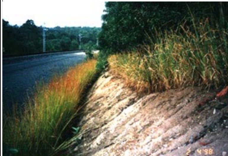
Australia: Railroad cutting stabilised by vetiver grass hedgerows. No other plant would grow on the cutting. As a result of the hedgerows the railroad bed drains no longer need extensive and costly annual cleaning -- Paul Truong
