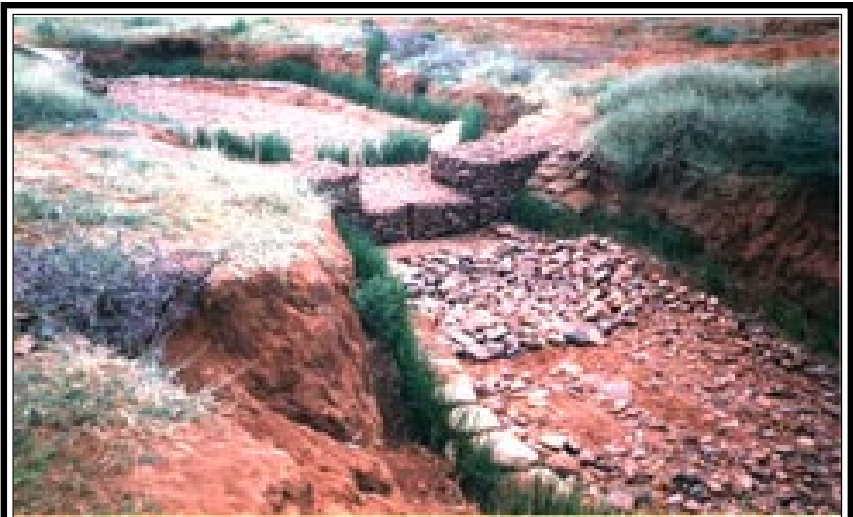
Zimbabwe: A roadside gully stabilized with rocks, gabions, and vetiver grass. Ultimately the rocks will be washed out leaving the vetiver grass as the prime means of protection. Photo Credit -- Stange Consult
