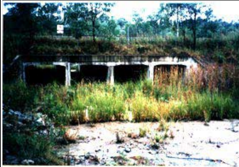
Australia: Railroad culvert stabilised by two lines of vetiver grass hedgerows both on the inlet side (to reduce sediments and therefore desilting costs) and on the outlet side to stop erosion and drainage floor cut back. Photo Credit -- Paul Truong
