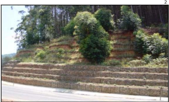
The view of the protected side slope demonstrating the combined use of gabion walls and the erosion control methods deployed have successfully achieved the required stability. Little or no silt deposits can be observed along the full extent of the concrete side drains.
