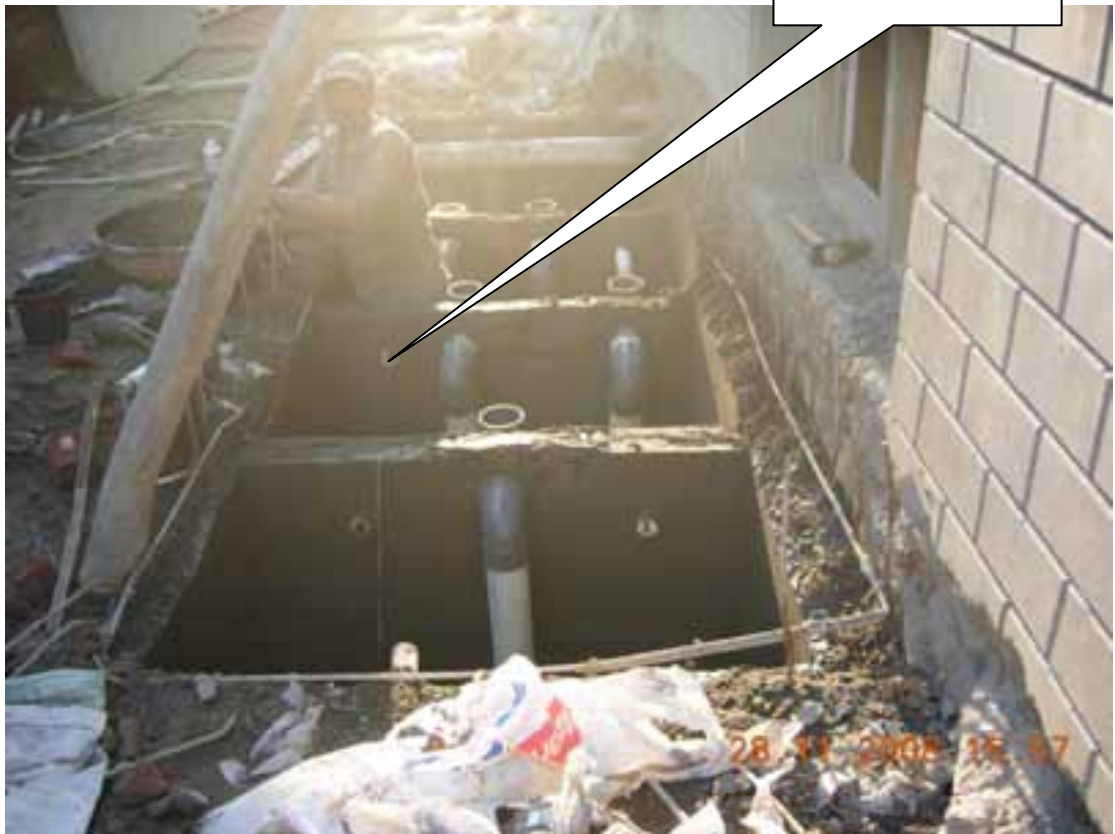
Four Chamber Baffled Reactor (Anaerobic)
