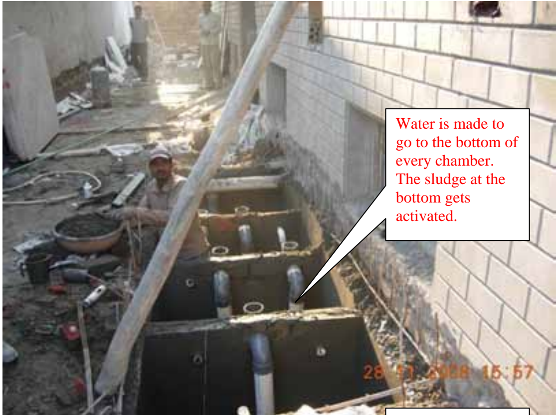
Four Chamber Baffled Reactor (Anaerobic)
