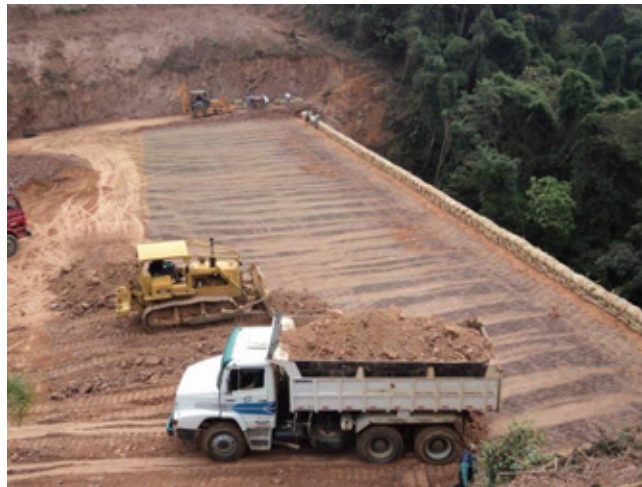
Filling site with soil
