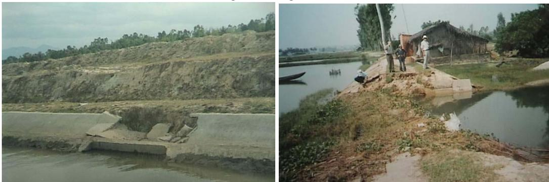
**Photos 3: Flood damages to asphalted road and farm road**
