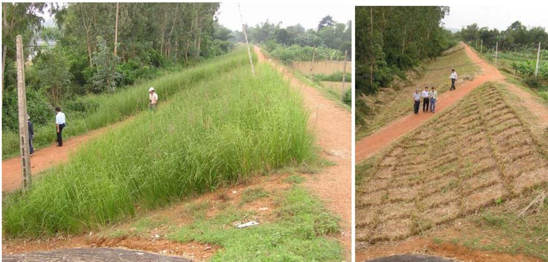
**Photo 7:** Drainage canal bank stabilisation, before and after vetiver planting
