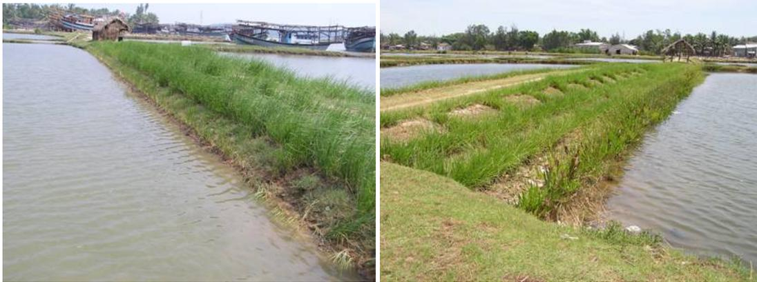
**Photo 5:** River bank stabilisation against flash flood erosion
