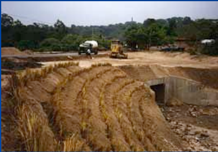
El Salvador - VS for bridge/culvert protection. Newly planted vetiver hedgerow
