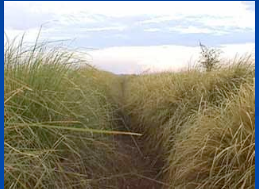
Madagascar - Vetiver stabilizes this irrigation canal
