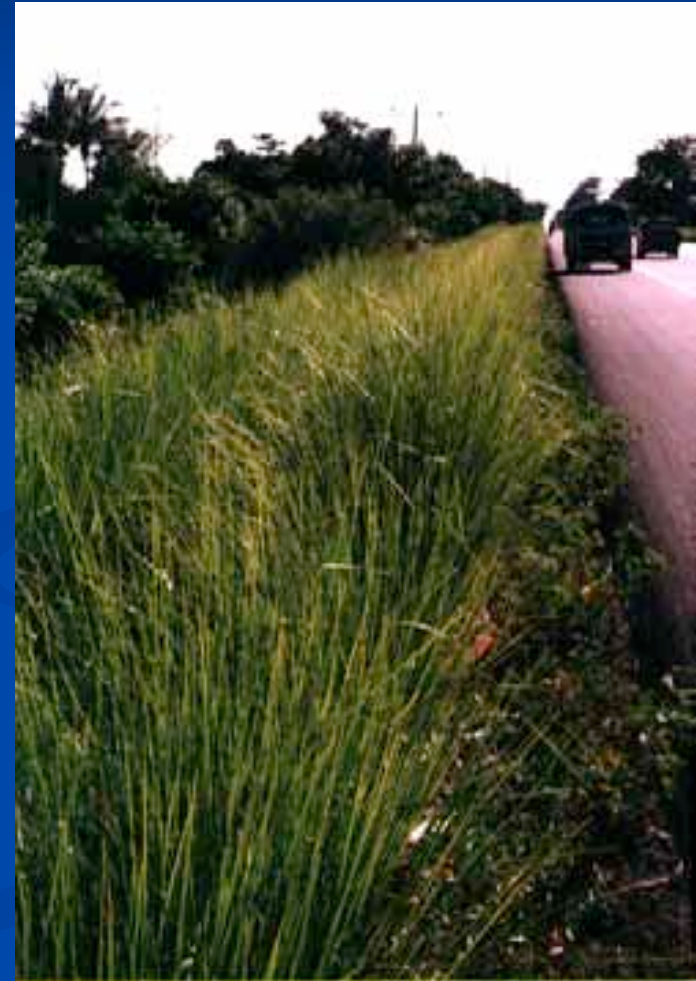
El Salvador - mature vetiver hedge protecting road embankment
