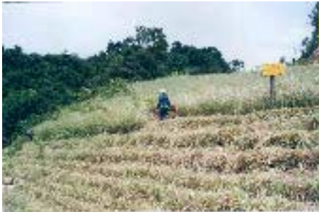
Figure 4 : KP 0+050, Trimming Vetiver Grass after the rainy season
