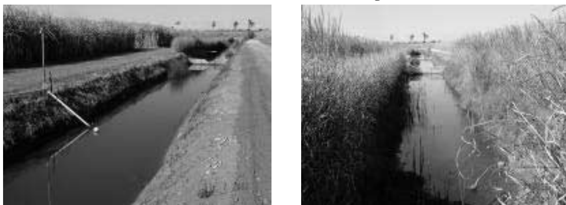
Photo 4 Exposed and highly erodible banks of the control section (left) as contrast to the well stabilised section of the trial (right)
