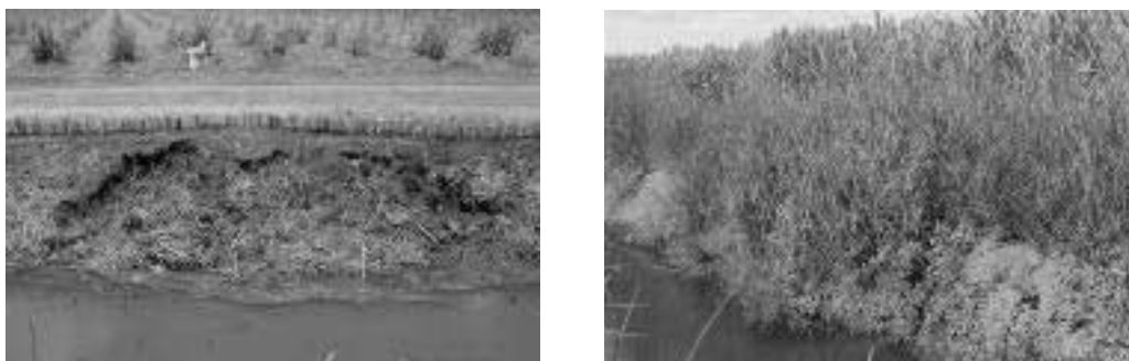
Photo 3 Vetiver was planted on this eroded section in November 2001 (left) and it was completely stabilised 6 months later (right)
