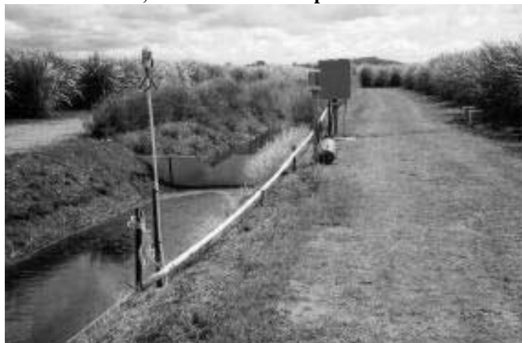
Photo 1 Multipoint Sensor Chamber mounted in electronics cabinet, pluviometer, pressure transducers, runoff and vetiver planted section weirs
