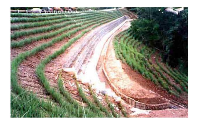
On this highway in Malaysia a major drainage section has been protected by planting a series of vetiver hedges, thus preventing, slips filling the drain and rendering it useless, these hedges will keep the road open during heavy tropical rain storms of over 5,000 mm annually. and prevent any slipping from the road fill. Thus saving hundreds of thousands of dollars in maintenance and keeping the road open for essential access to markets and infrastructure.
