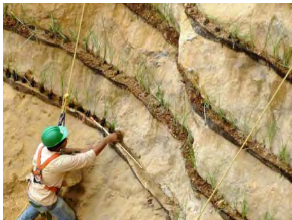
Ambitious vetiver project, vertical stabilization
