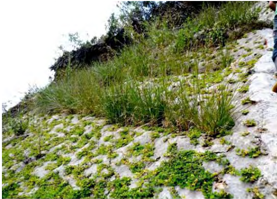
Eco mortar with Vetiver terraces and Pinto Peanut groundcover
