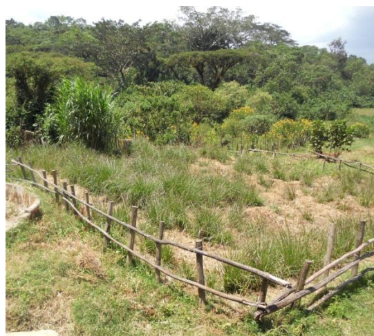
Figure 6: The wetland is lumpy, missing vetiver plants, and the slope is uneven.
