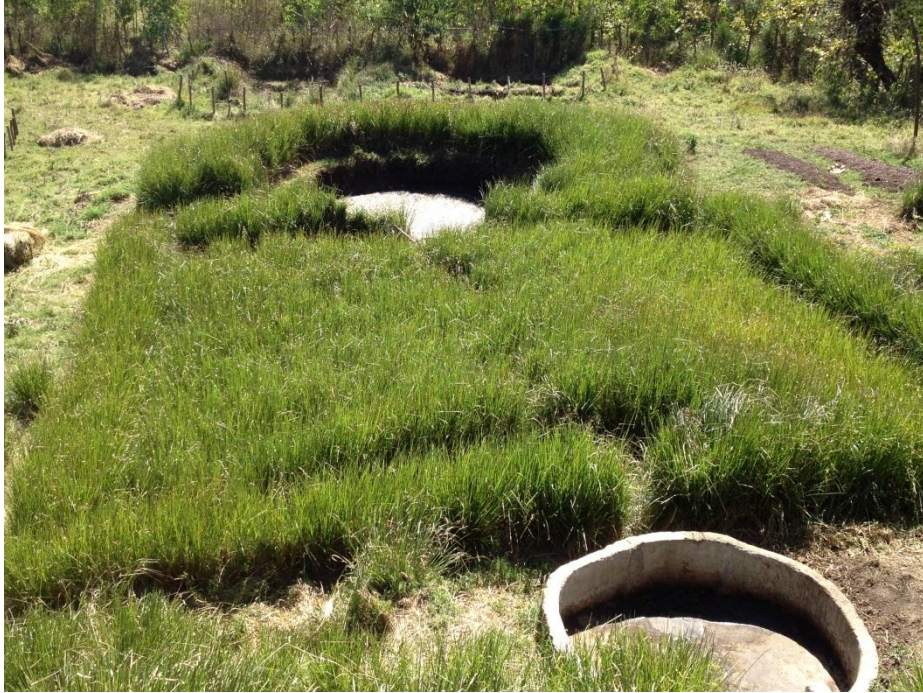
Figure 9: Established vetiver wetland ready for the season to start. The pulp retention basin is seen in the bottom right corner and the evaporation pond with concentric circles of vetiver is at the top of the picture.
