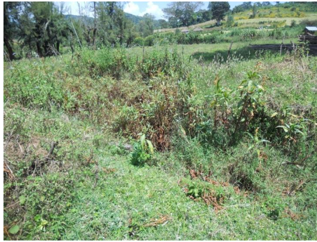
Figure 7: The evaporation pond full of tall weeds.
