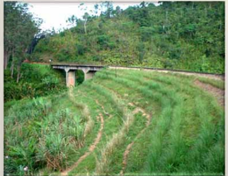
Railroad bridge batter protection
