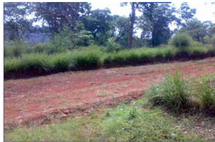
Fig. 6. Vetiver used to stabilize
