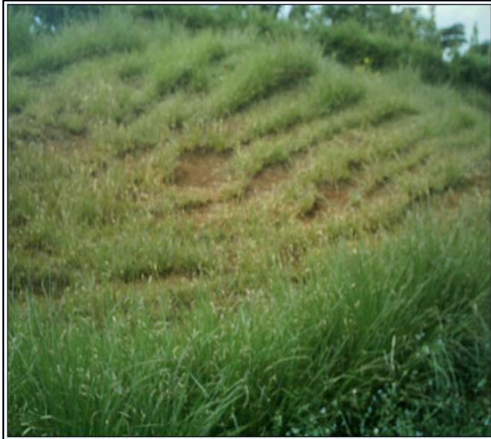
Fig. 7. Vetiver hedge rows used to stabilize the fill up/ cut soil at pulping stations in CPDE.
