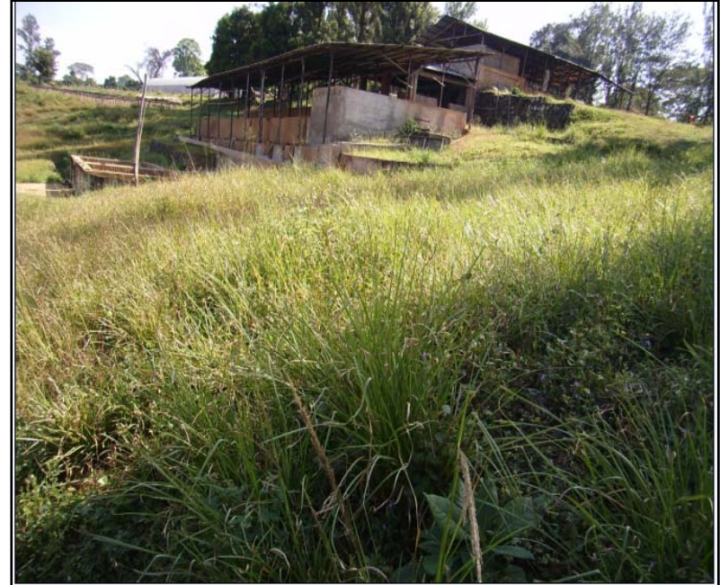
Fig. 7. Vetiver hedge rows used to stabilize the fill up/ cut soil at pulping stations in CPDE.
