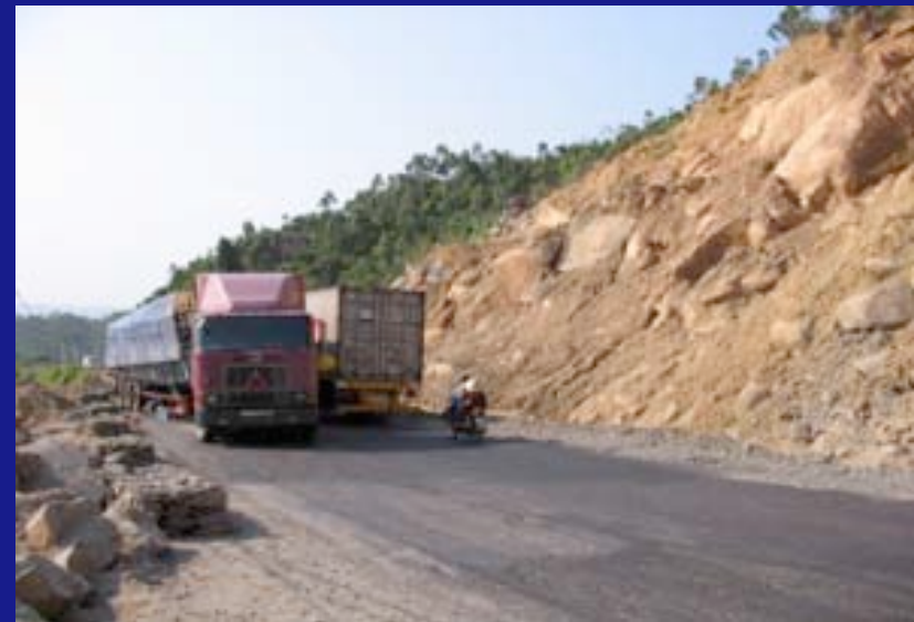
This cut (left) was not stabilized and slipped (right) blocking traffic)
