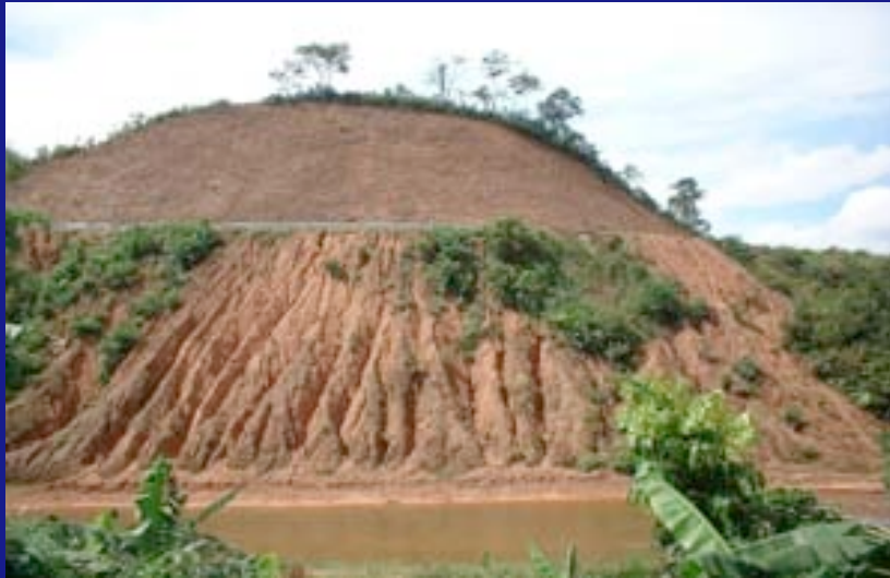
Unprotected highway fill (left) ends up in the nearby river (right), polluting the water supply of thousands downstream users.
