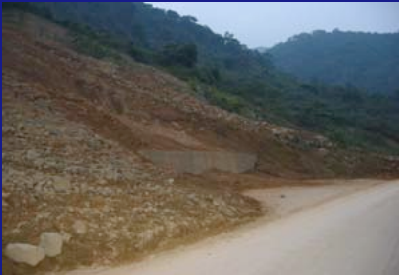
This cut (left) was not stabilized and slipped (right) blocking traffic)
