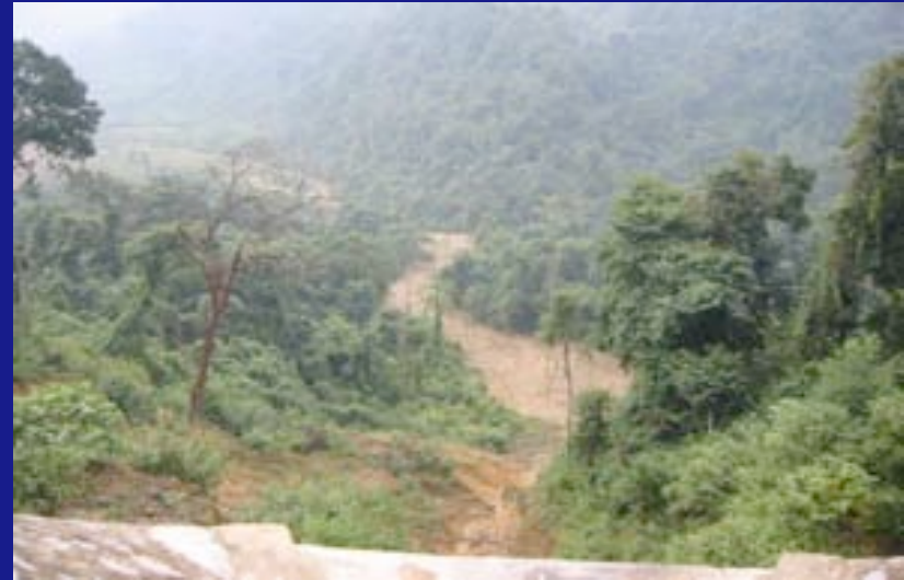
Unprotected highway fill (left) ends up in the nearby river (right), polluting the water supply of thousands downstream users.
