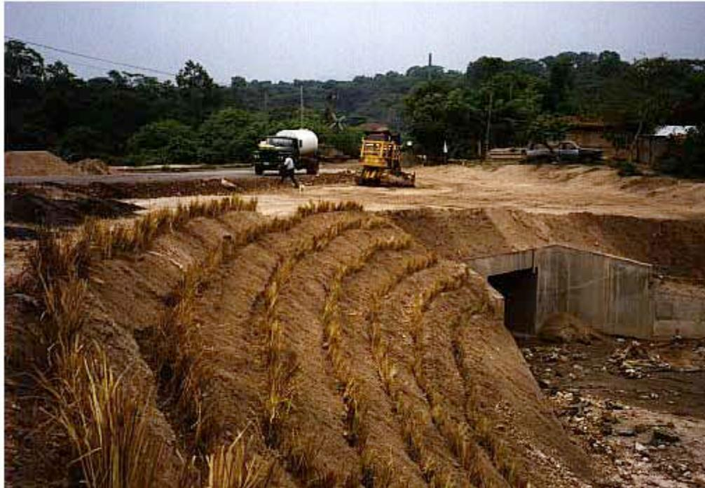
El Salvador This type of VS protection at the fill /culvert interface is essential if road washouts are to be avoided at the time of heavy flooding
