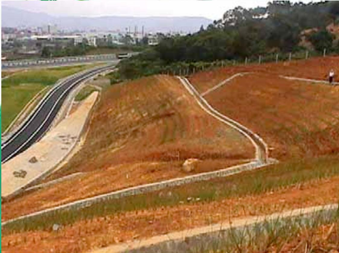
China Cut slopes such as these can be stabilized with VS (actually vetiver has just been planted here)
