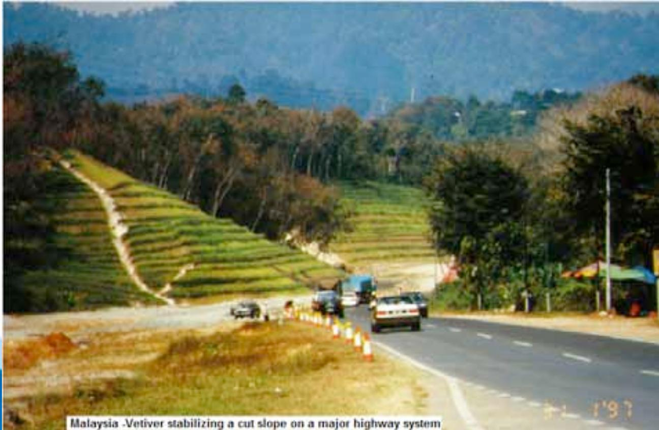
Malaysia - Vetiver stabilizing a cut slope on a major highway system
